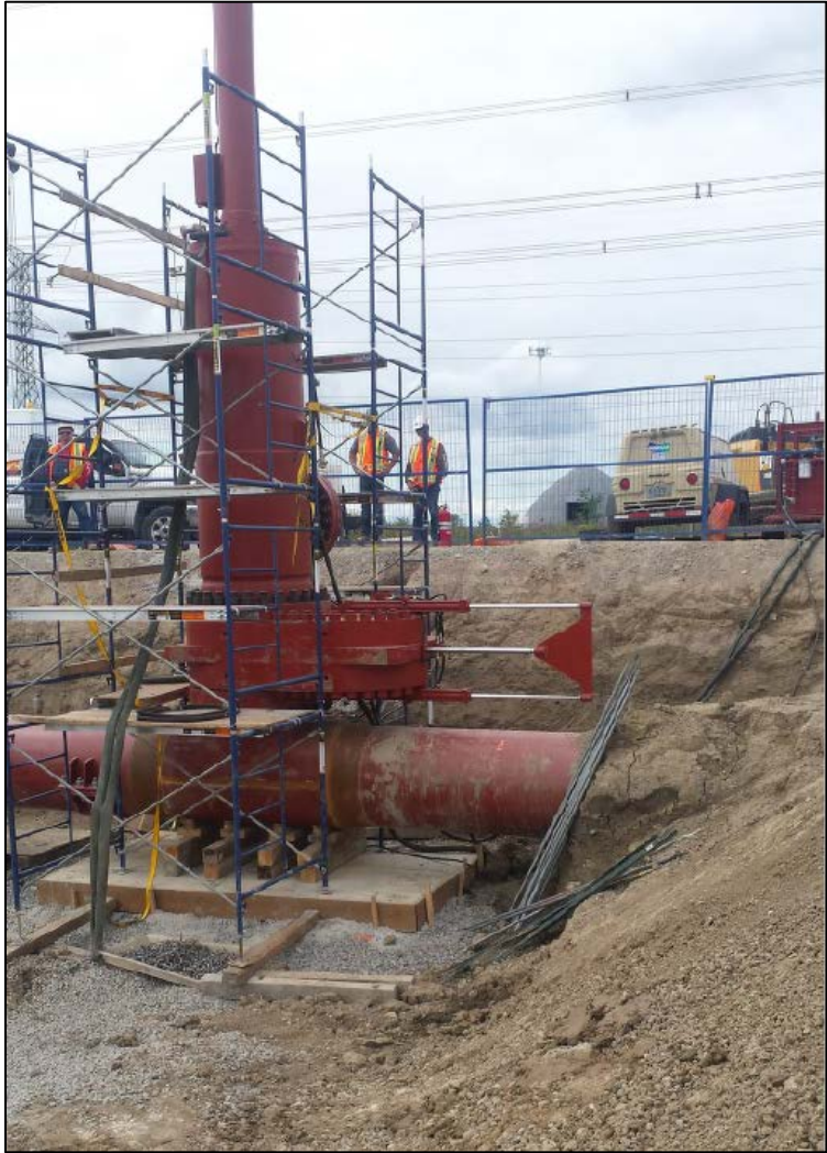
Figure 1: Stopple Fitting
