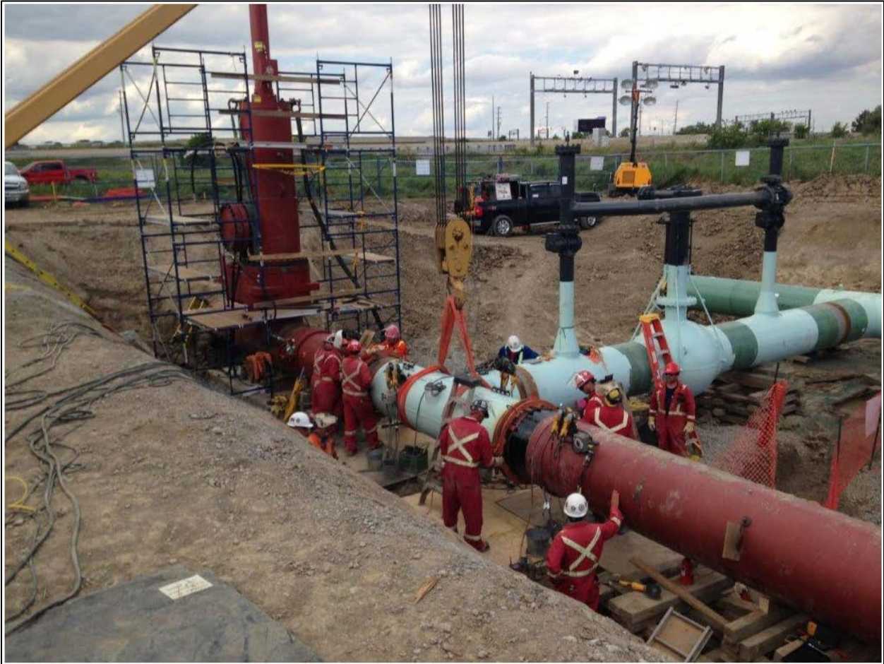
Figure 4: Typical Working Area and Stopple Fitting on Parkway North NPS 36
