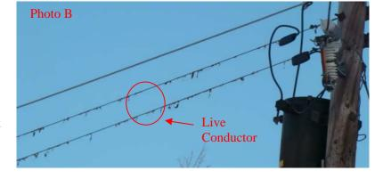
secondary bus is approximately 30 to 40 years old. The insulation has decayed and fallen off exposing the energized copper conductor (See Photo B). In some cases the exposed copper conductor has come in contact with each other in adverse weather conditions creating arcing seen from the street level, resulting in call outs of line personal. Innisfil plans to replace the open wire secondary bus with an insulated aluminum triplex bus.
