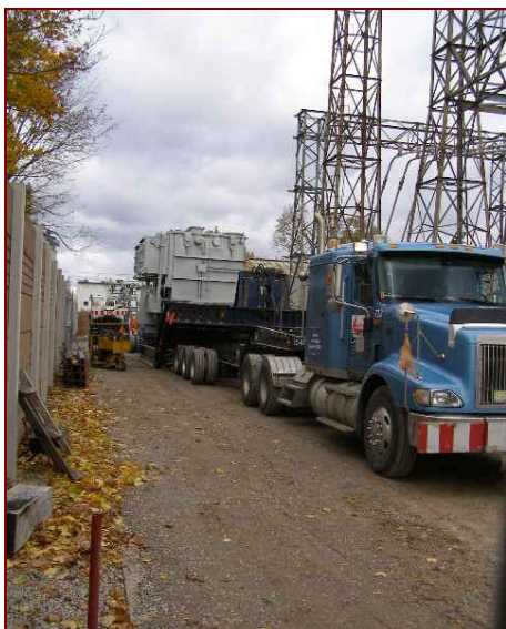
Fig 2 – Truck delivering new transformer
