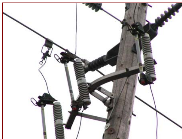
Figure 15, Non-insulated bracket at 5093 (2K2)
