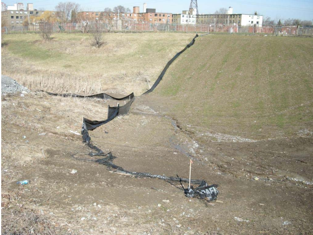
Photo 17 –Tie-in point at Jonesville District Station (sediment fencing to be repaired)
