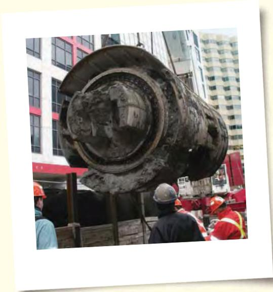
In 2006, Hydro One completed digging a 2.2-kilometre tunnel beneath the streets of Toronto. This innovative project will carry an array of electricity transmission lines to tie the east and west halves of the city together, with minimal disruption to traffic or residents. Expanding the links between east and west by running new transmission lines through the \$45 million investment will let power flow more freely across the city, giving Toronto increased flexibility, reliability and supply.
