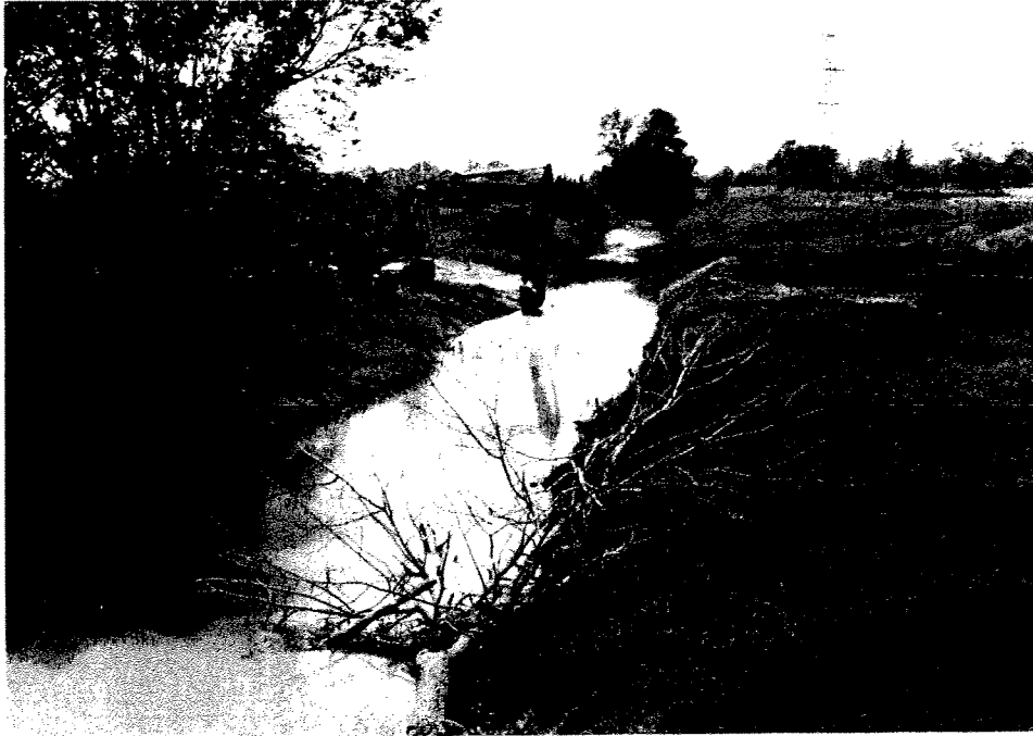
Photo 3: Clay Creek banks and bottom being restored to final shape by CATERPILLAR hoe in June, 1990.
