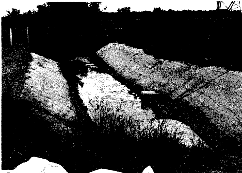
Photo 6: Erosion control matting used to stabilize banks of municipal drains.
