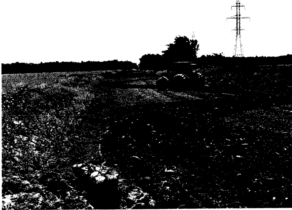
Photo 1: Chisel ploughing of easement. Note the "S" shape of initial ploughing pattern.
