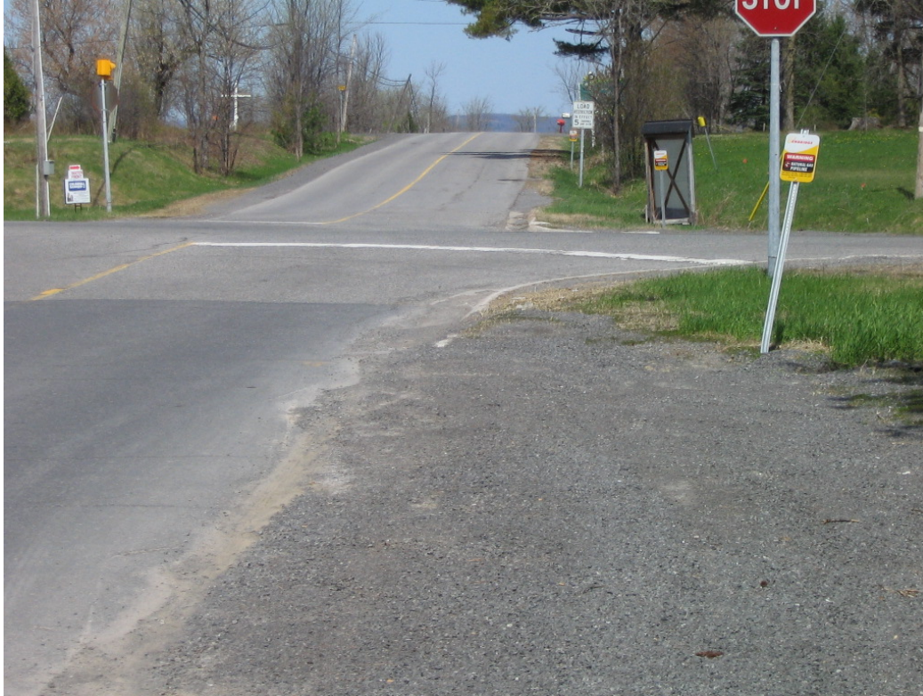
Photo 13 – Looking north; County Road 26 at Highway 17
