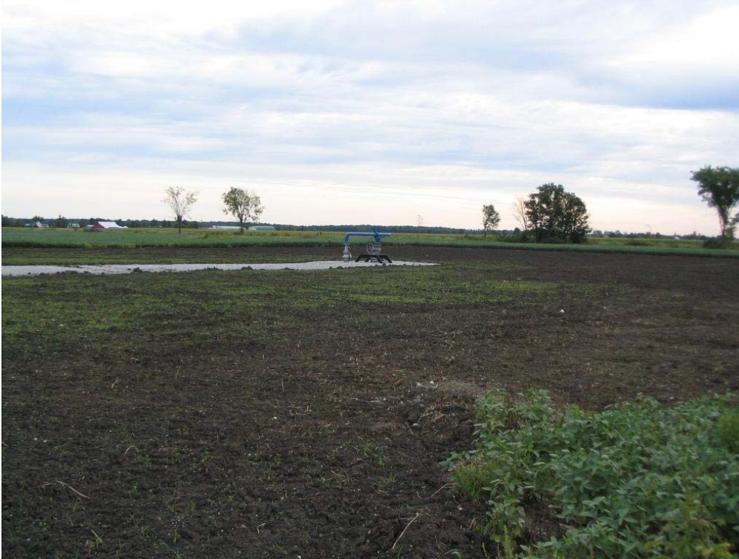
Photo 3: Looking northeast; topsoil replaced
