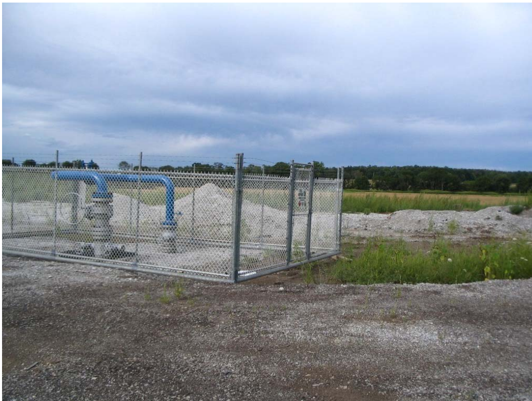
Photo 2 – TW#13H; looking southwest
