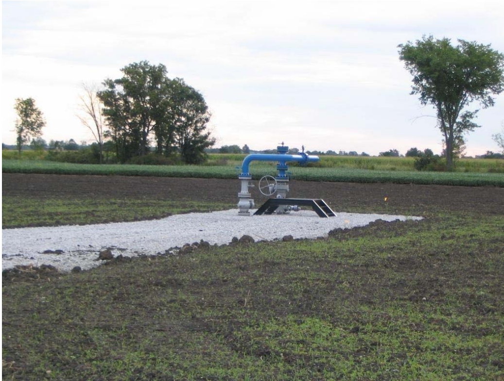
Photo 1 – TKC#61H looking northeast
