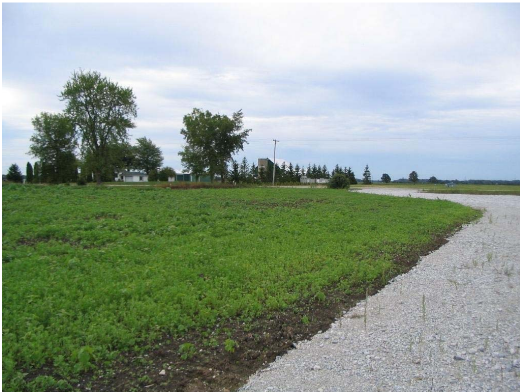
Photo 4: Looking southeast towards Moore Road; Access Road
