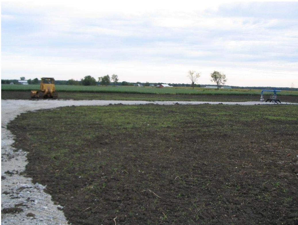
Photo 2 – Looking north; topsoil replaced
