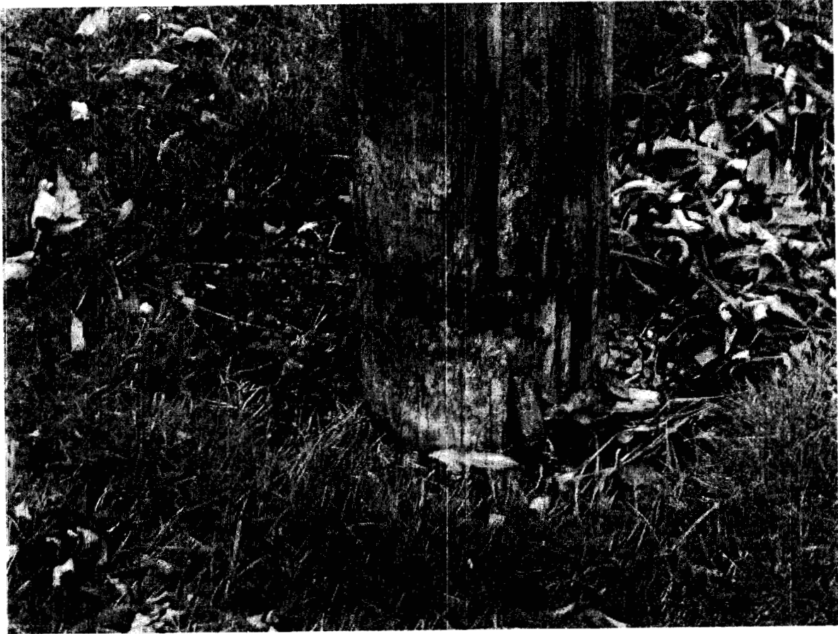
Pole Rotting at Base
