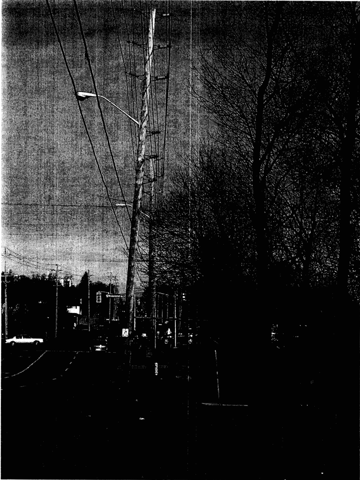
Leaning Pole Caused by Slack Guy (across the road)
