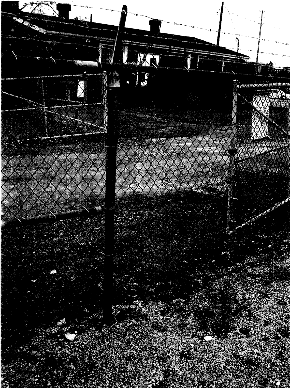
Missing (stolen) Station Fence Ground
