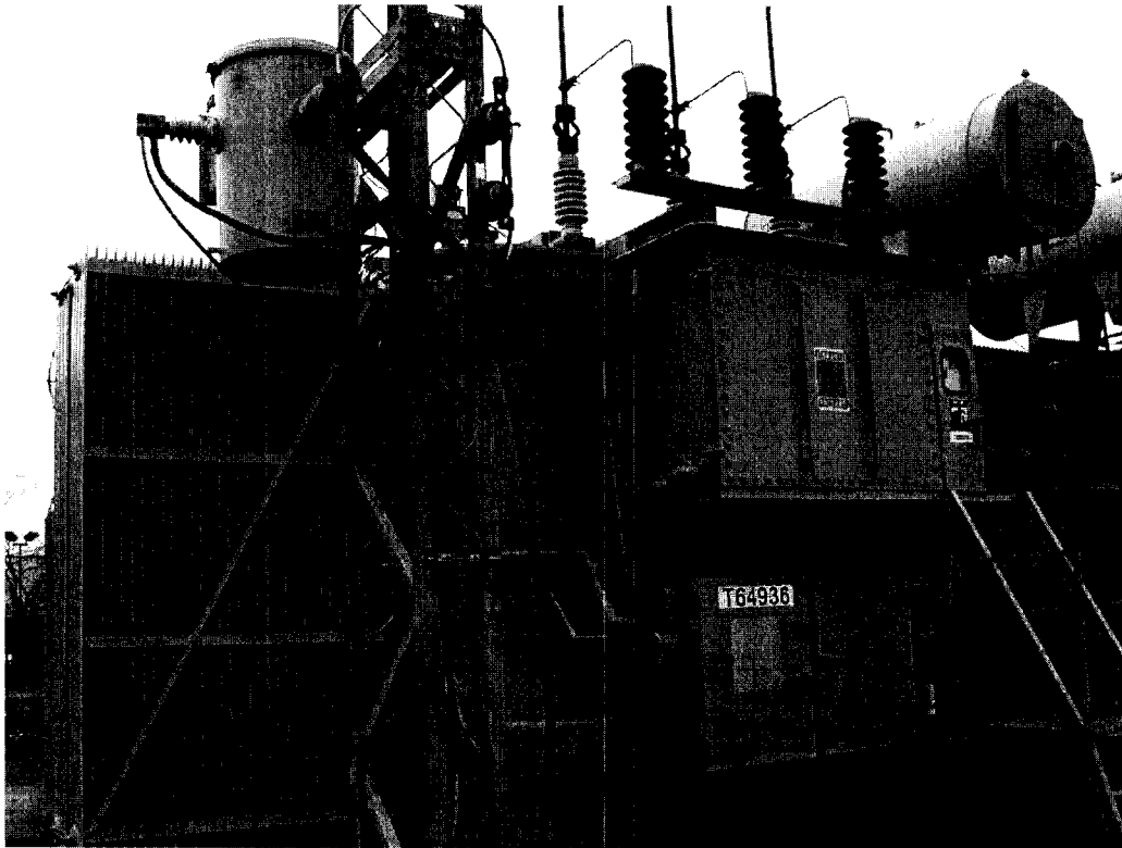
Well Maintained Older Transformer
