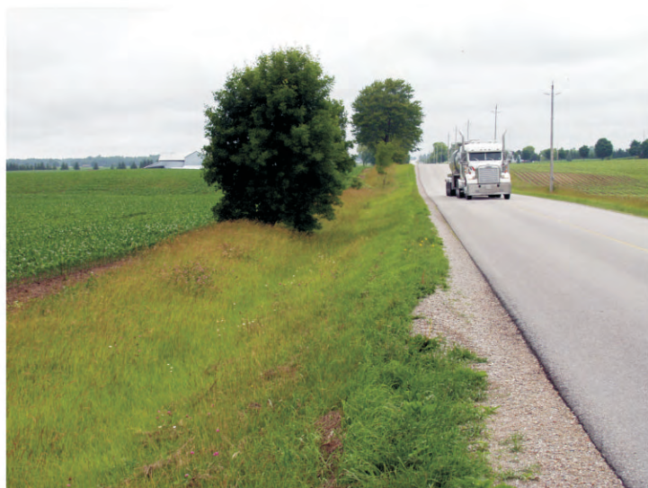
Plate 14 Goshen Line between Huron Street and Kirkton Road, View North
