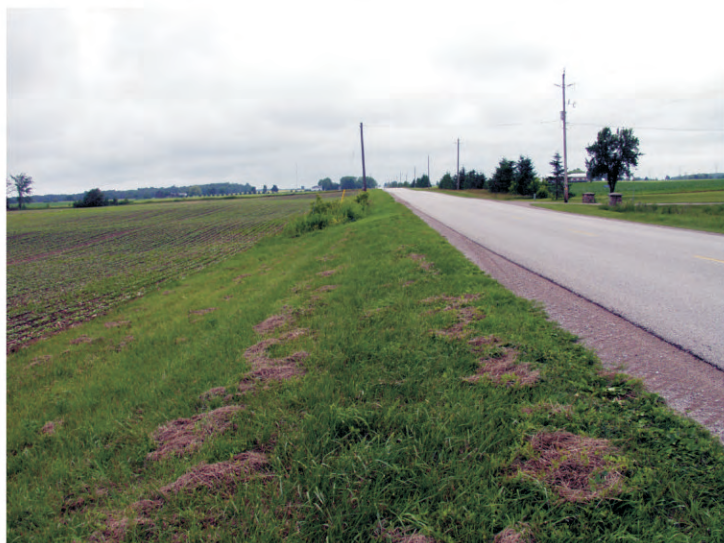
Plate 13 Goshen Line between Dashwood Road and Huron Street, View North
