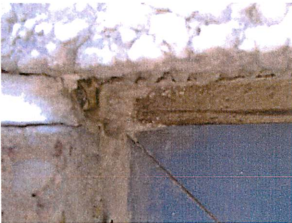
Caulking failures at window to precast
