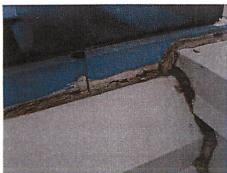
Condition found at the 2 nd floor, south west corner between the window, the precast and the roof parapet flashing.
