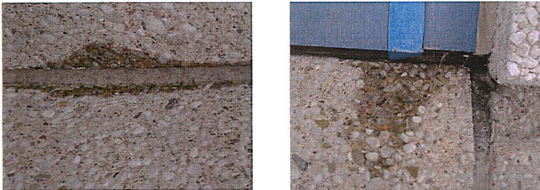
Evidence of moisture trapped within the caulked cavities weeping through the joint between the caulking and the precast. Note that I had not rained for a few days.
