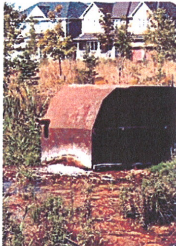
MINERALIZED WATER FROM SEWER CONSTRUCTION STAINS THE GROUND RED AS IT FLOWS TO A ROUGE TROUT STREAM (SEPTEMBER, 2003).
