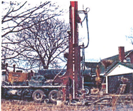
RURAL WELL DEEPENING CANNOT KEEP UP WITH THE AQUIFER DRAWDOWN CAUSED BY THE YORK DURHAM SEWER CONSTRUCTION DE-WATERING.
