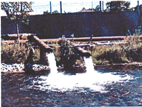
MASSIVE YORK-DURHAM SEWER CONSTRUCTION DEWATERING OF ORM AQUIFERS BESIDE ROUGE STREAM.
