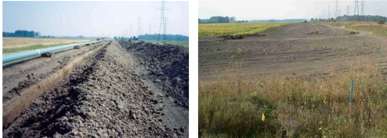
Installation of a 20" diameter pipeline before and after pipeline installation
