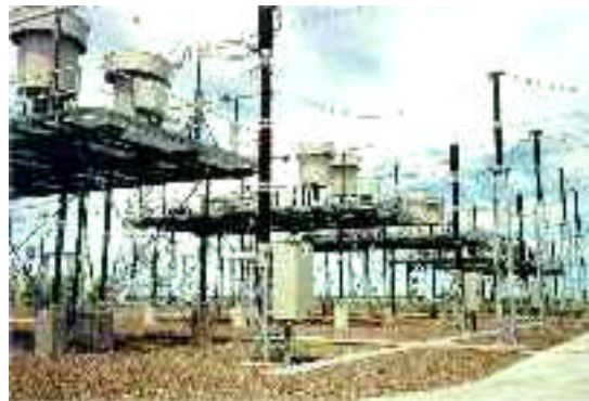
Fig. 14: 500 kV series capacitors.
