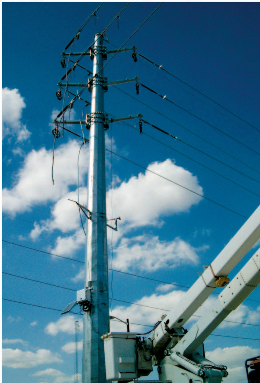
Deadend structure for ACCR test line. Note the installation of the CAT-1 system and weather instrumentation below the conductors.
