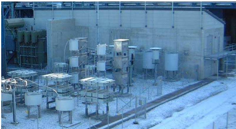
STATCOM – Synthesize AC from DC
