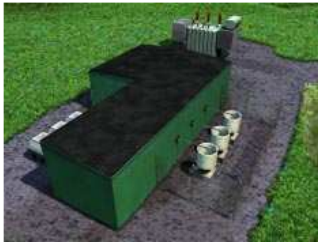
Fig.15 : Typical SVC Light for utility applications.
