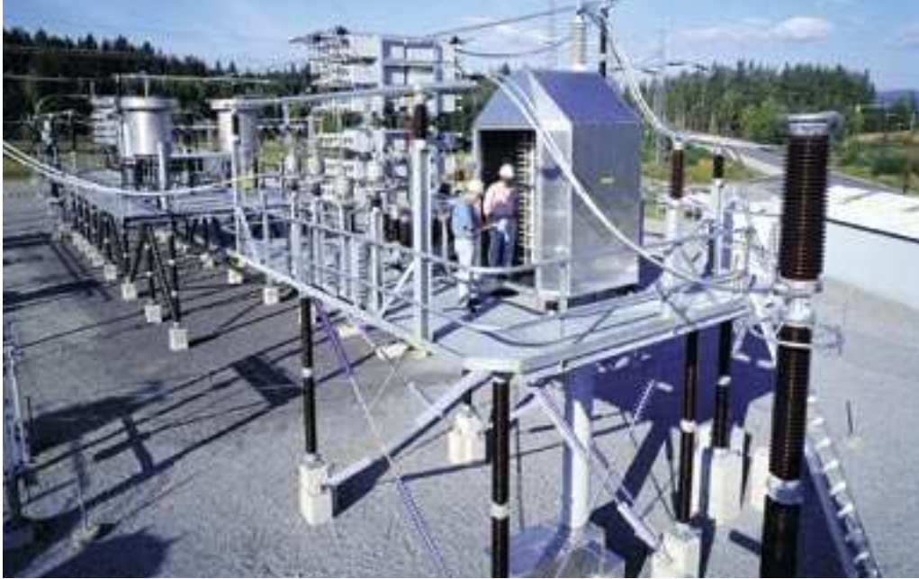
Thyristor-controlled segment of a series capacitor.
