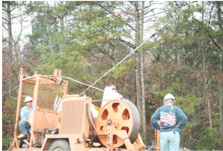
Figure 3- Bull wheel tension of conductor during installation
