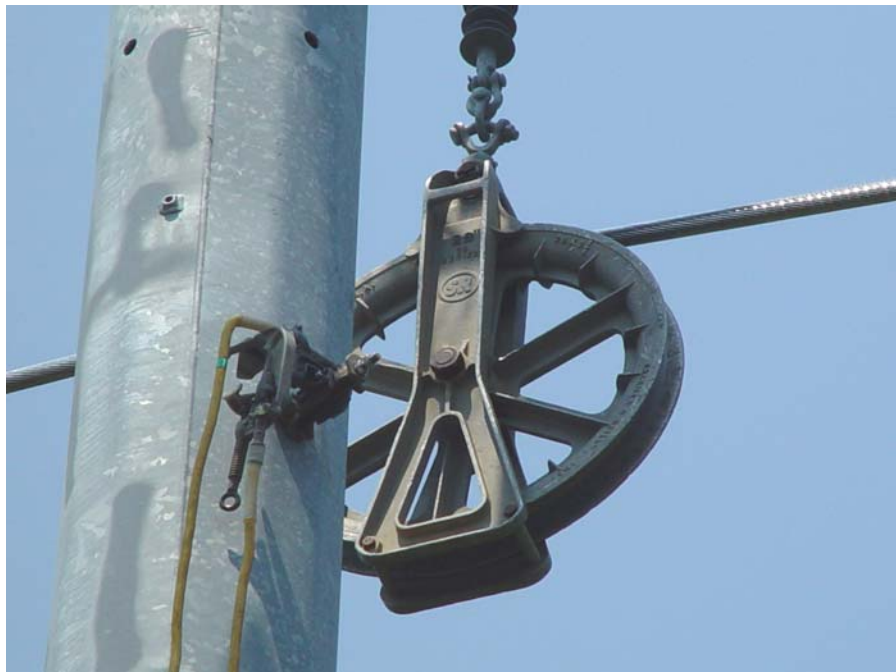
Figure 2- Sheave used in the installation
