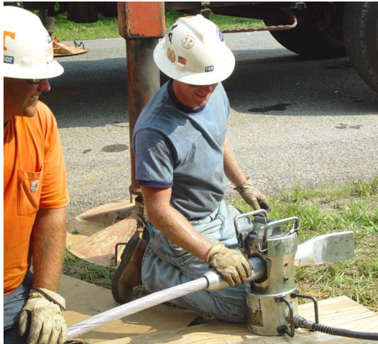
Figure 6- Compression of jumper connector
