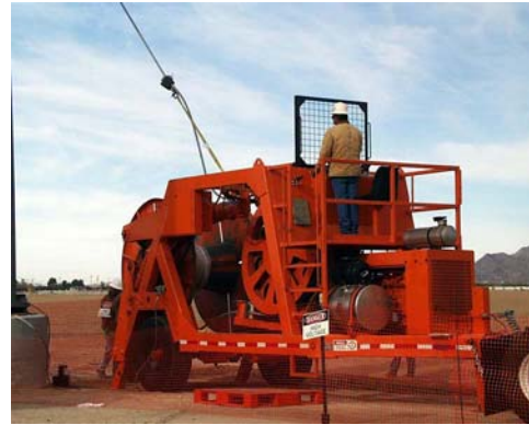
Figure 5 – Puller (Tensioner)
