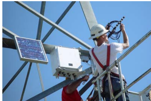
CAT-1 system installed on the line
