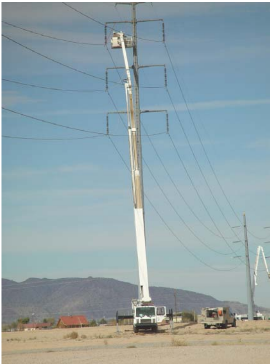
Installation of PLP THERMOLIGN™ Suspensions
