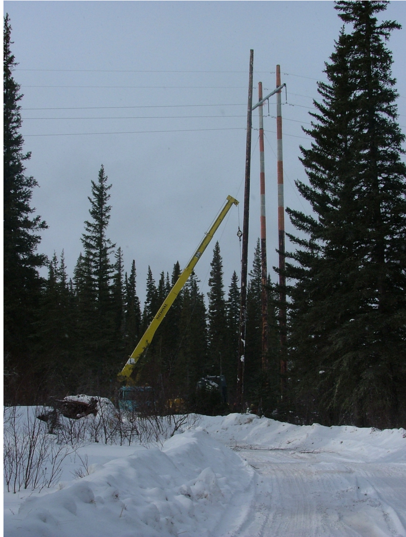
Workers setting a pole for the Lawashi River crossing, south of Attawapiskat. The ADSS pole line parallels the existing transmission line.
