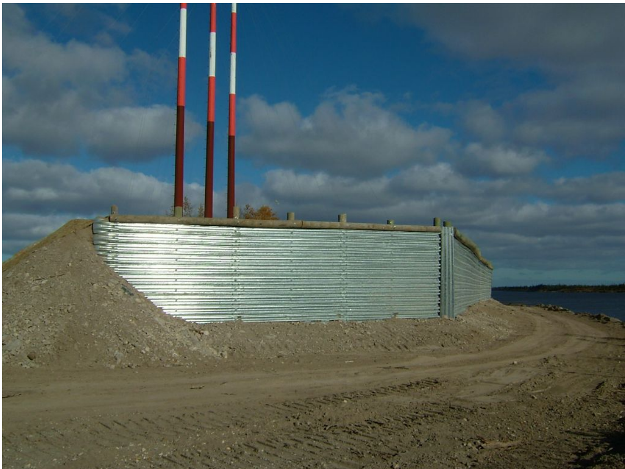
4 5 Newly constructed ice berm wall protecting structure 909 on north side of the Albany River
