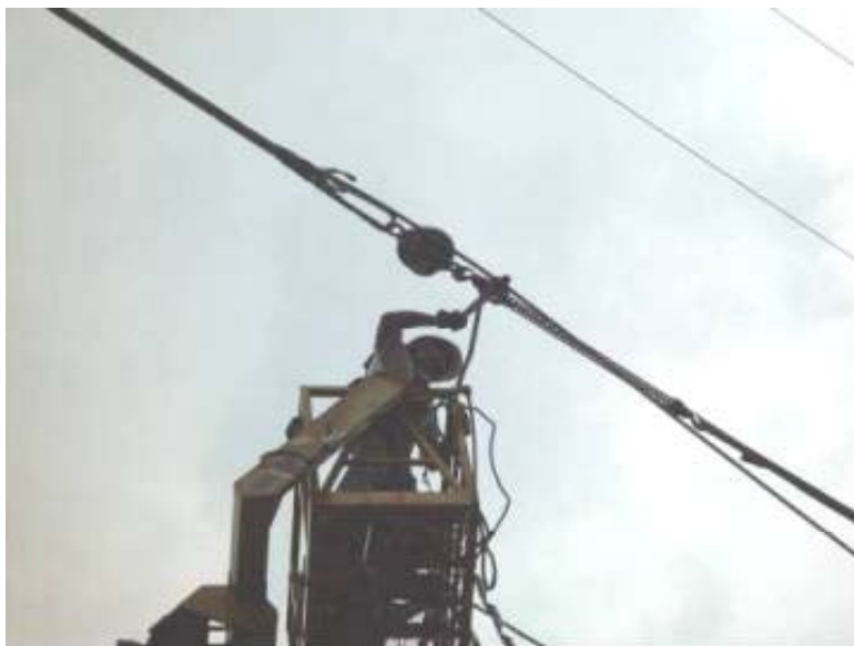
Figure 4- Sagging with chain hoist and dynamometer
