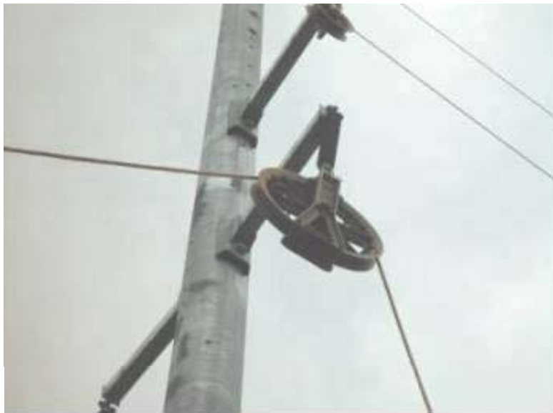
Figure 3- Conductor stringing
