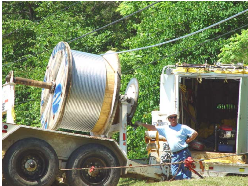
Figure 5 Conductor unwinding station
