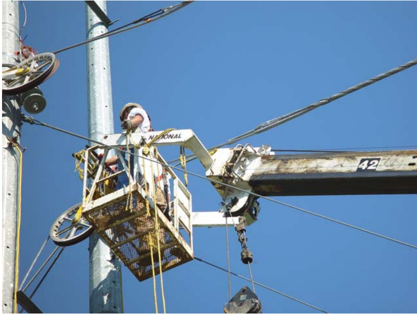
Figure 2 PLP dead end installation using double 28” sheave at the first tower
