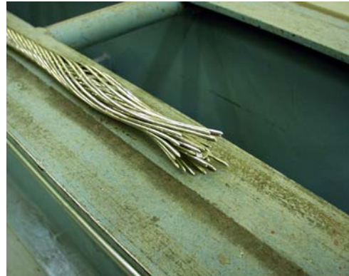
Figure 2 – Typical Mid-Span Failure
