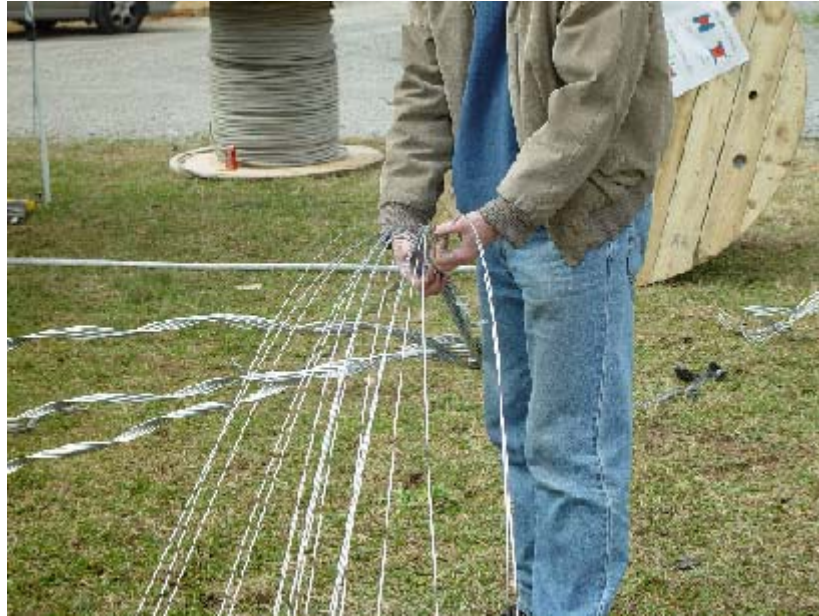
Figure 5. Undamaged Conductor core wires after sheave testing.
