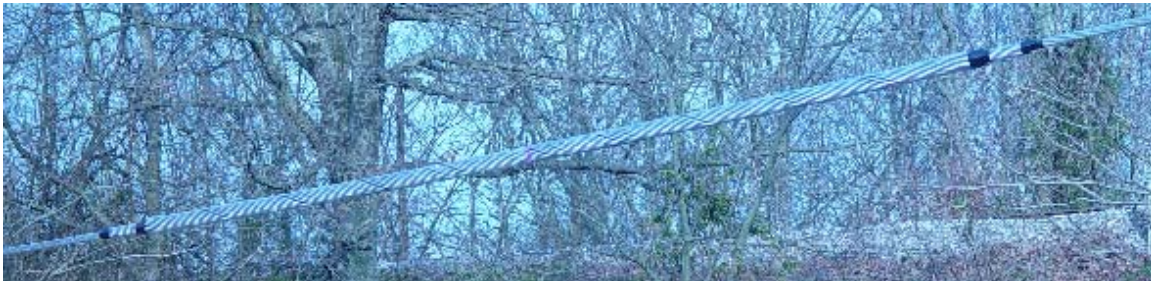
Figure 3. Fully configured splice in the test loop
