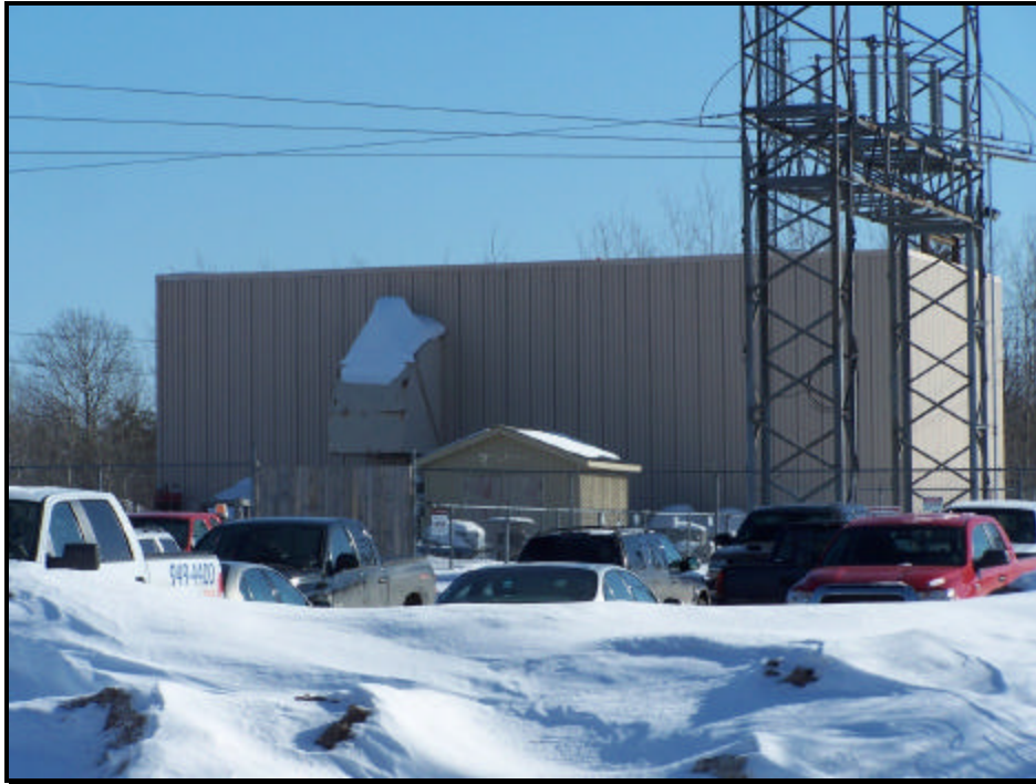
Side View of Storage Building
