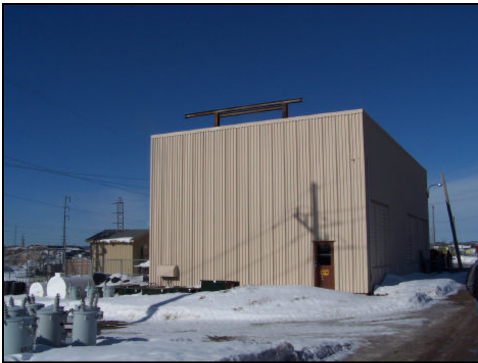
Rear View of Storage Building
