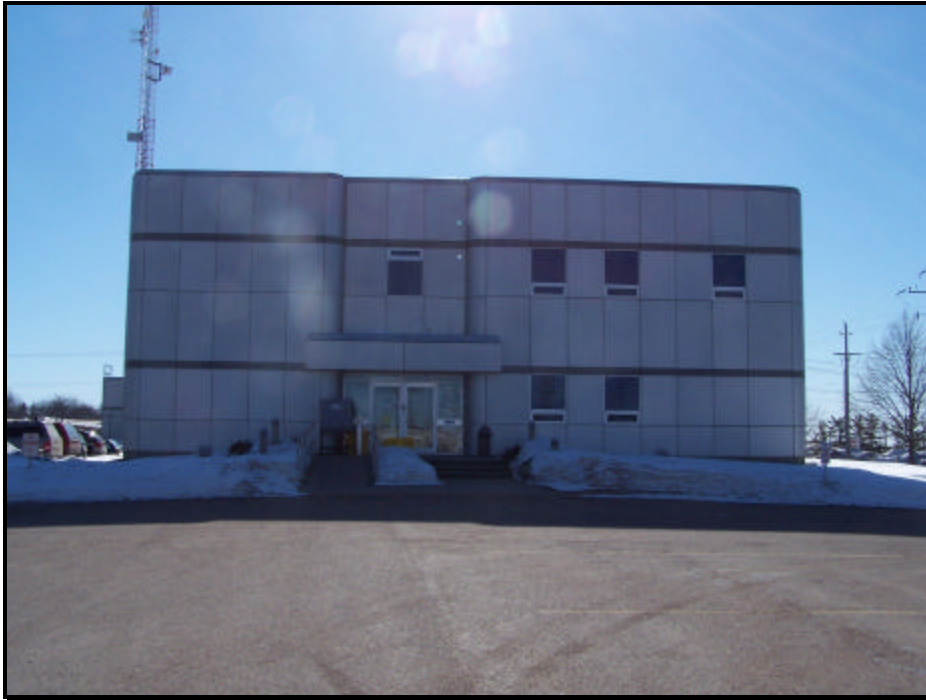
Front View - 2 Storey Portion
