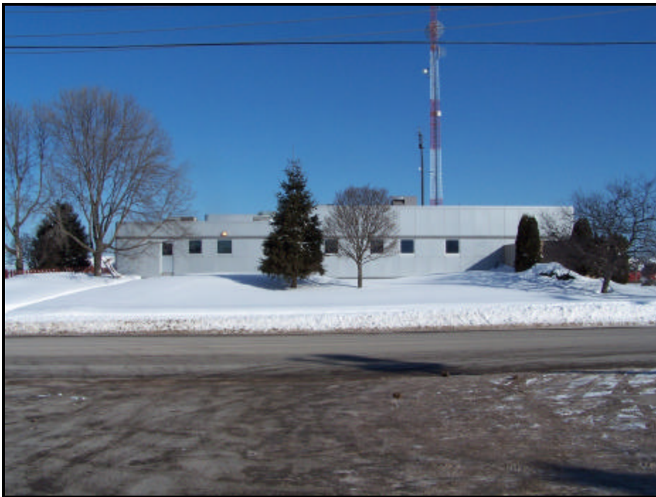
Rear View - One Storey Portion
