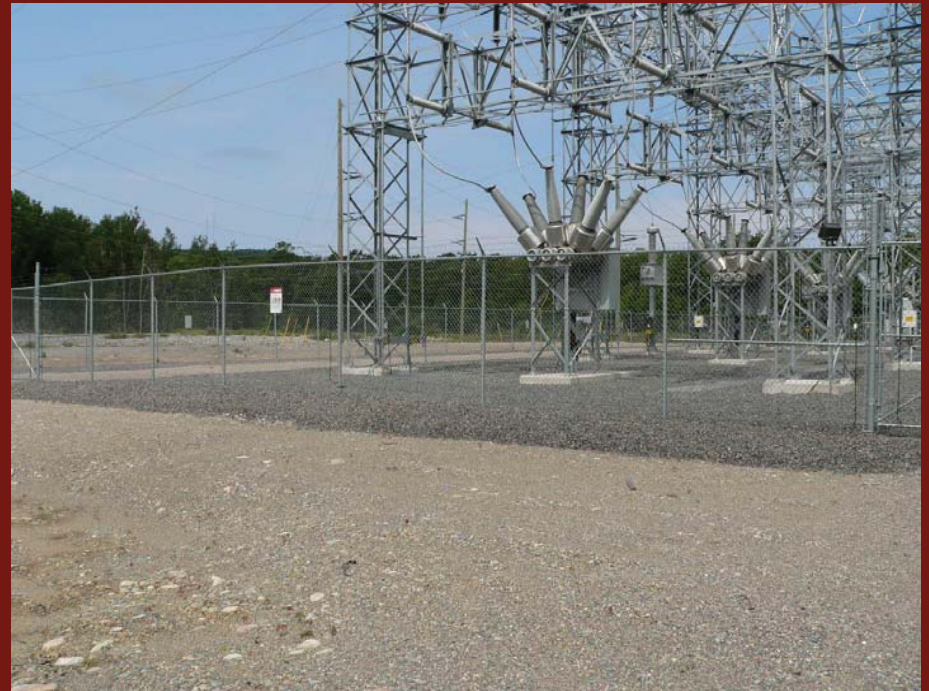
Figures 9 & 10 – Adequate crushed stone and ground grid mats as shown at Gartshore TS.
