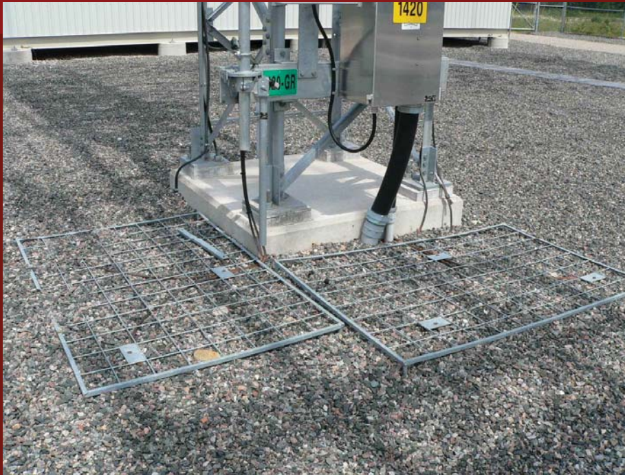
Figures 9 & 10 – Adequate crushed stone and ground grid mats as shown at Gartshore TS.
