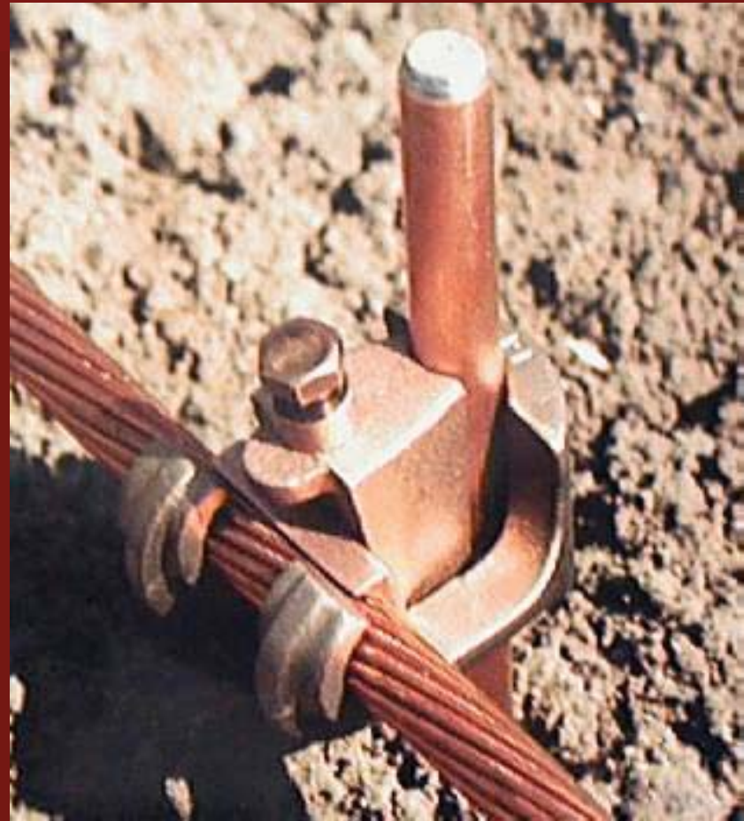
Figure 1 – Ground Grid Connection
