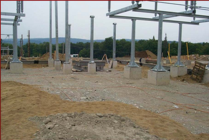
Figure 7 & 8 – Ground Grid Installation at Mackay TS 2008
