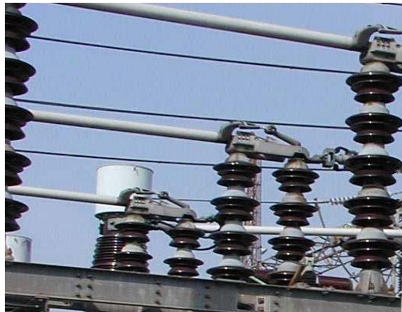
Figure 16: Station Cap and Pin Insulators
