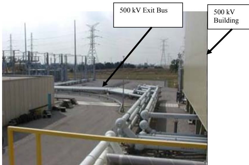
Figure 5: 500 kV GIS Outdoor Exit Bus Equipment
