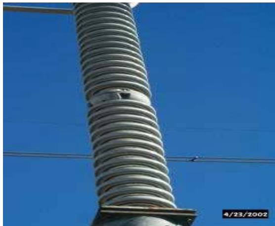
Figure 15: Station Porcelain Post Insulator
