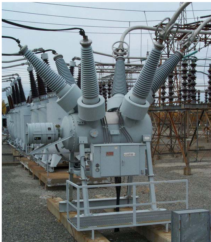
Figure 2: Dead Tank SF 6 Circuit Breaker
