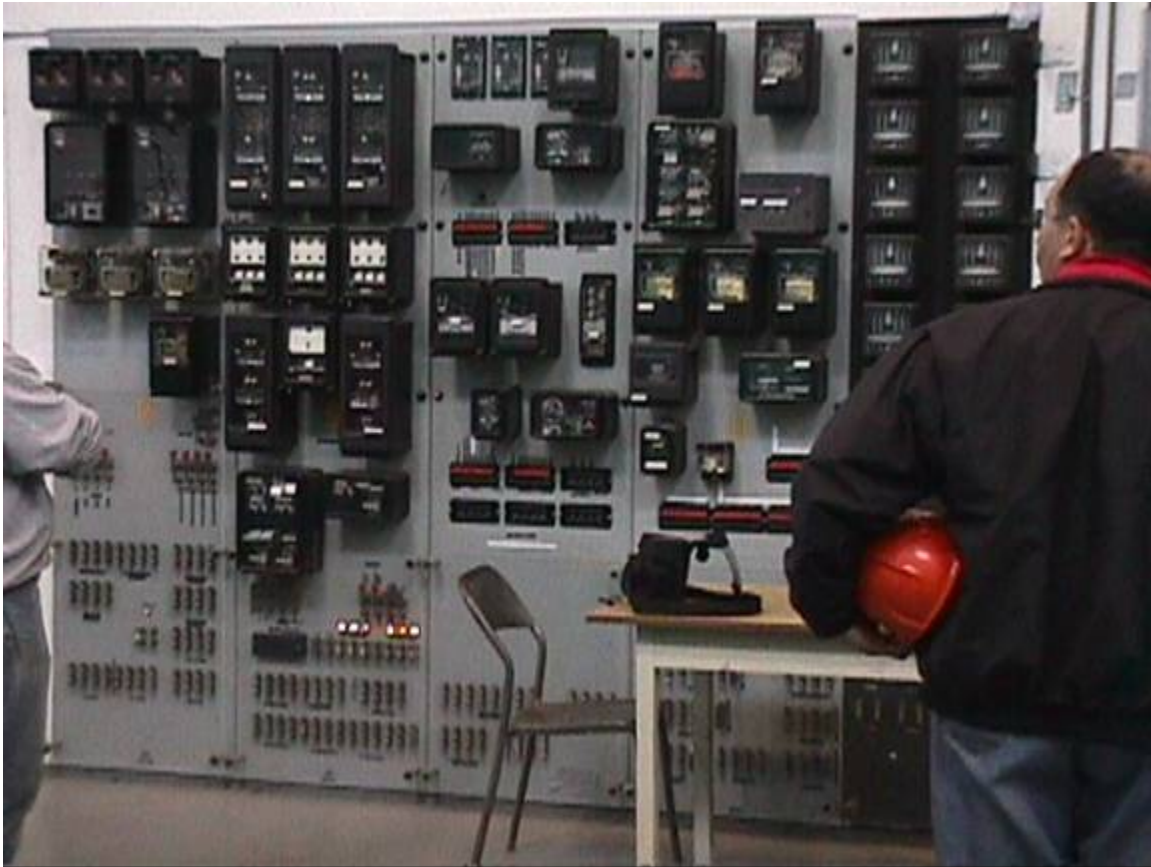
Figure 50: 24 Inch Steel-Type Panels with Protection, Auxiliary Relays, Flexitest Switches and Current Links
