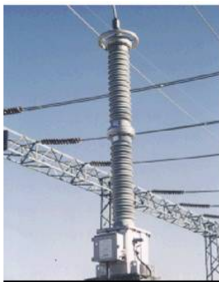
Figure 14: Capacitive Voltage Transformer
