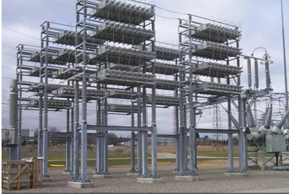
Figure 17: Capacitor Bank
