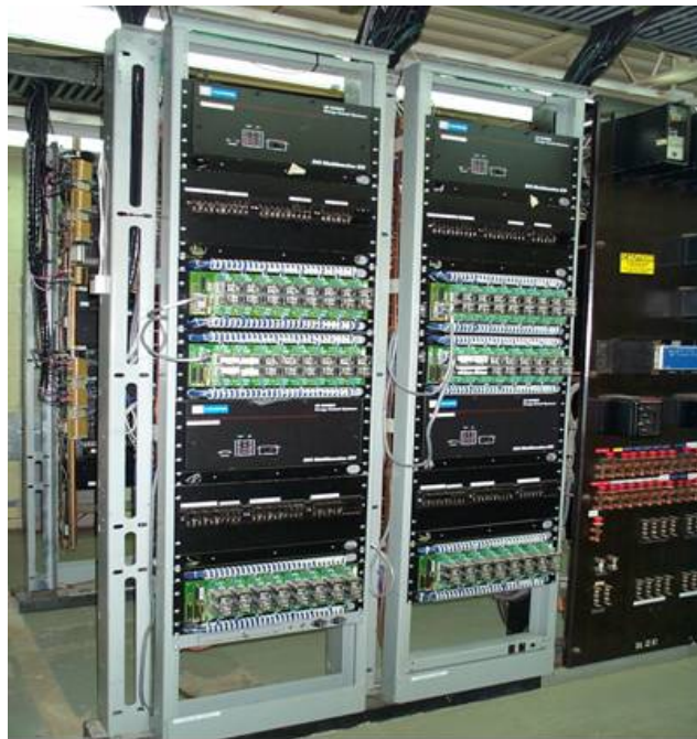
Figure 51: GE D25 Distributed RTU Installation - 1999
