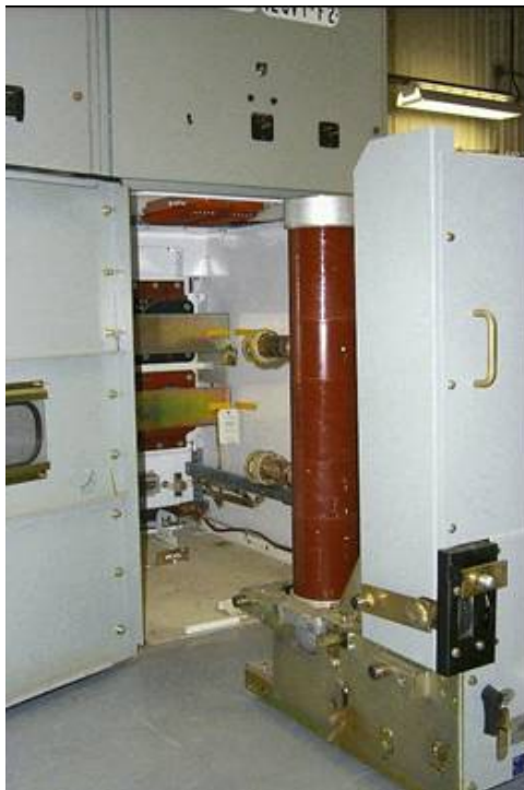
Figure 7: Circuit Breaker Withdrawn from Breaker Compartment
