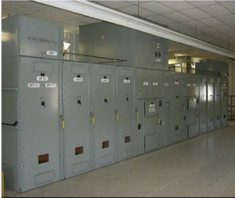
Figure 6: Typical Hydro One Metalclad Switchgear
