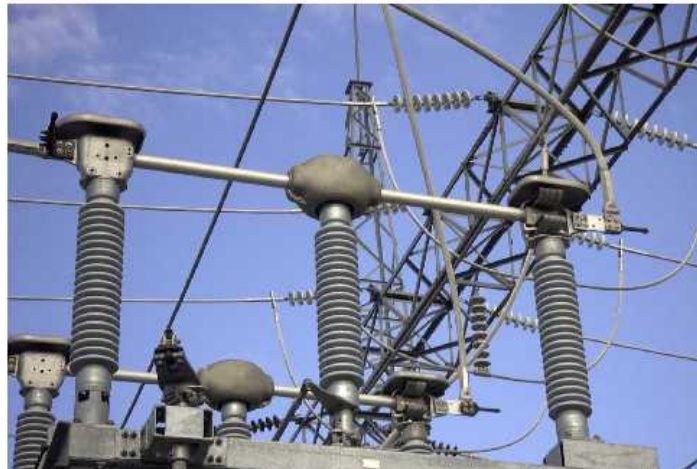
Figure 12: Center Rotating Disconnect Switch
