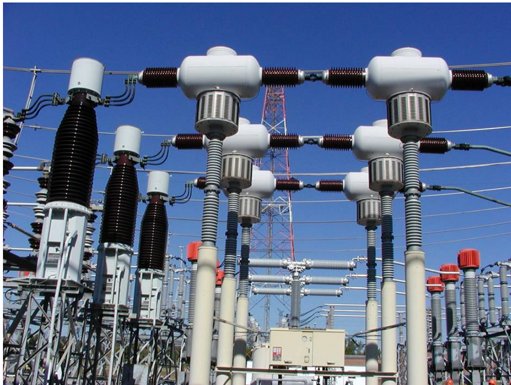
Figure 3: 230 kV Air Blast Circuit Breaker
