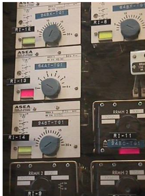
Figure 49: ASEA RR Type Auxiliary Relays
