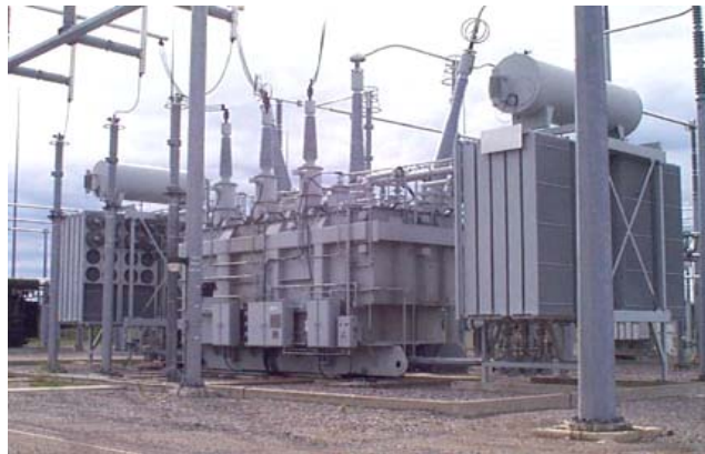
Figure 9: Typical Transmission Station Power Transformer
