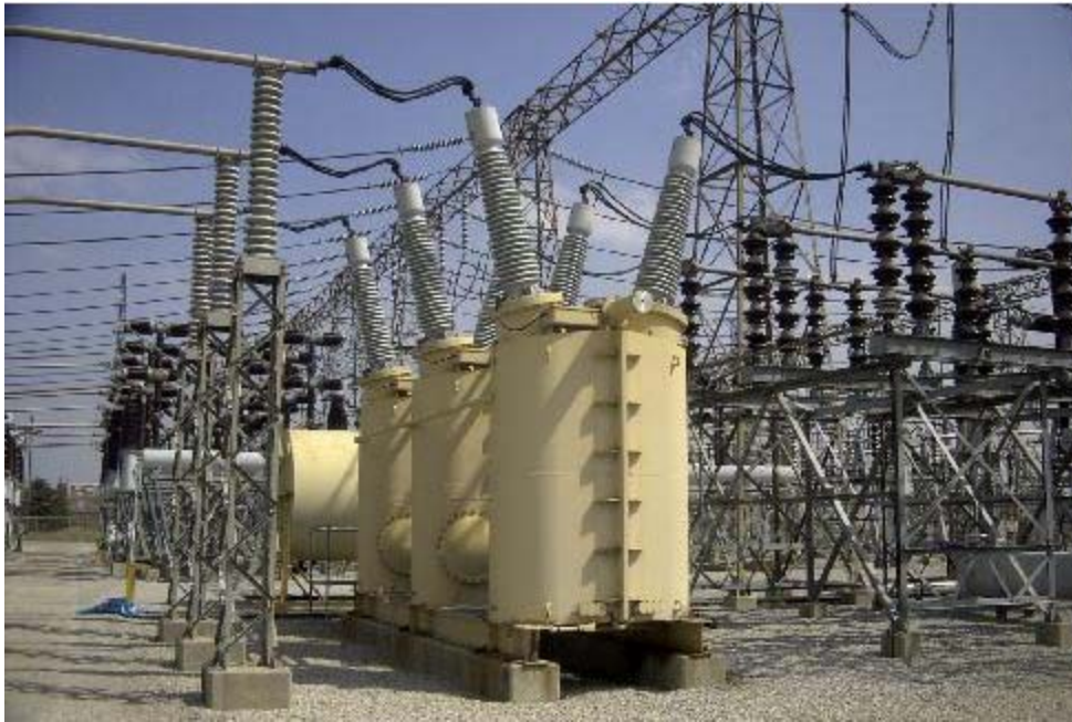
Figure 1 - Three Tank Oil Circuit Breaker
