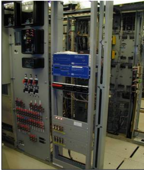
Figure 47: Digital Primary Schweitzer Relays
