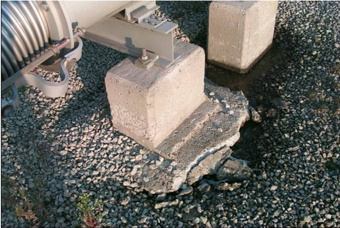
Figure 24: Damaged Footing of a SF 6 Bus Duct
