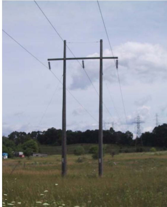
Figure 57: Transmission Line H-Frame Structure
