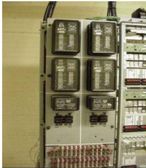
Figure 45: Electromechanical Relay Panel
