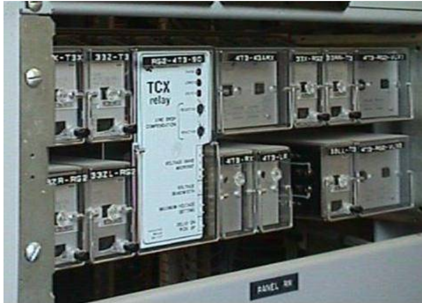
Figure 48: ASEA RX Type Auxiliary Relays
