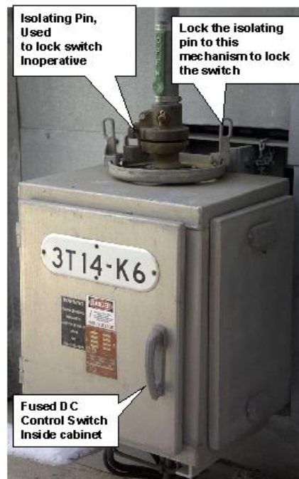
Figure 13: Motor Operating Mechanism for a Switch
