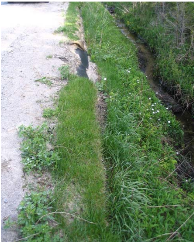
Photo 14 – Wilson Drive; bank erosion at headwater stream crossing
