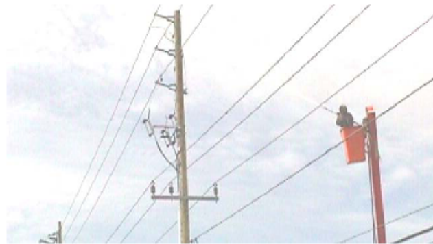
Washing older style porcelain line post insulator to reduce tracking and flashover
