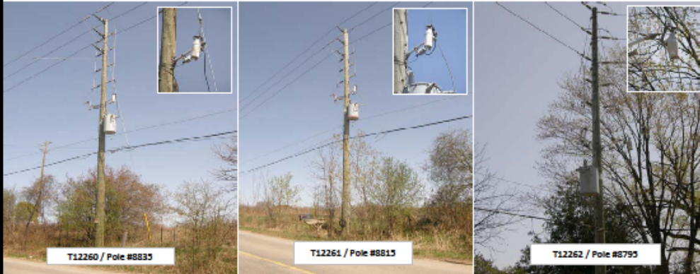
Installed Trip Saver Reclosers at Creditview Rd South of Queen St
