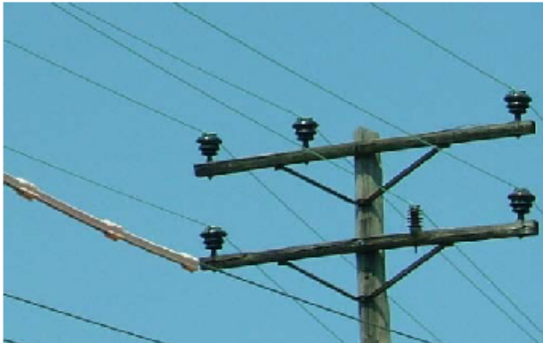
Older style pin type porcelain insulator
