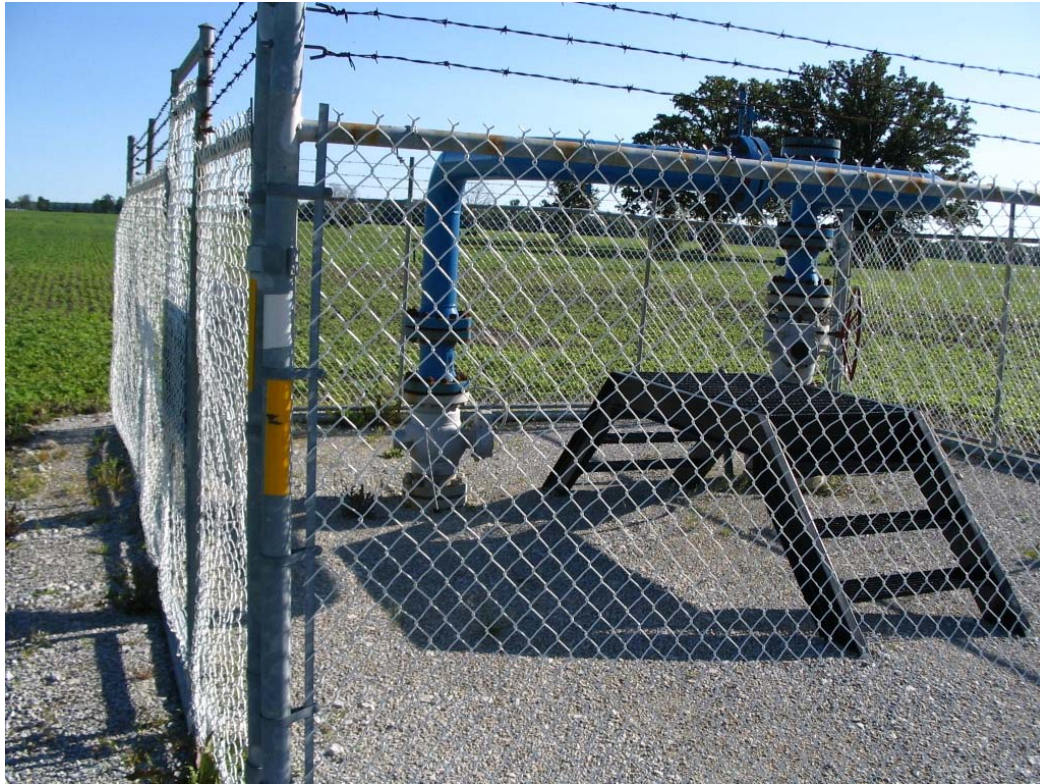
Photo 3: Looking north; west side of well
