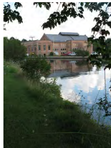
Healey Falls Generating Station
