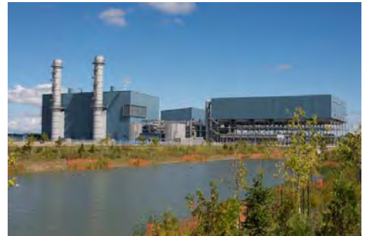
Halton Hills Generating Station
