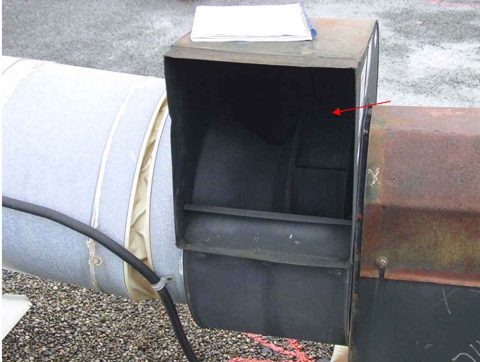
Photograph 17: Roof Area 1.1 – Existing exhaust openings lack protective rain hoods.
