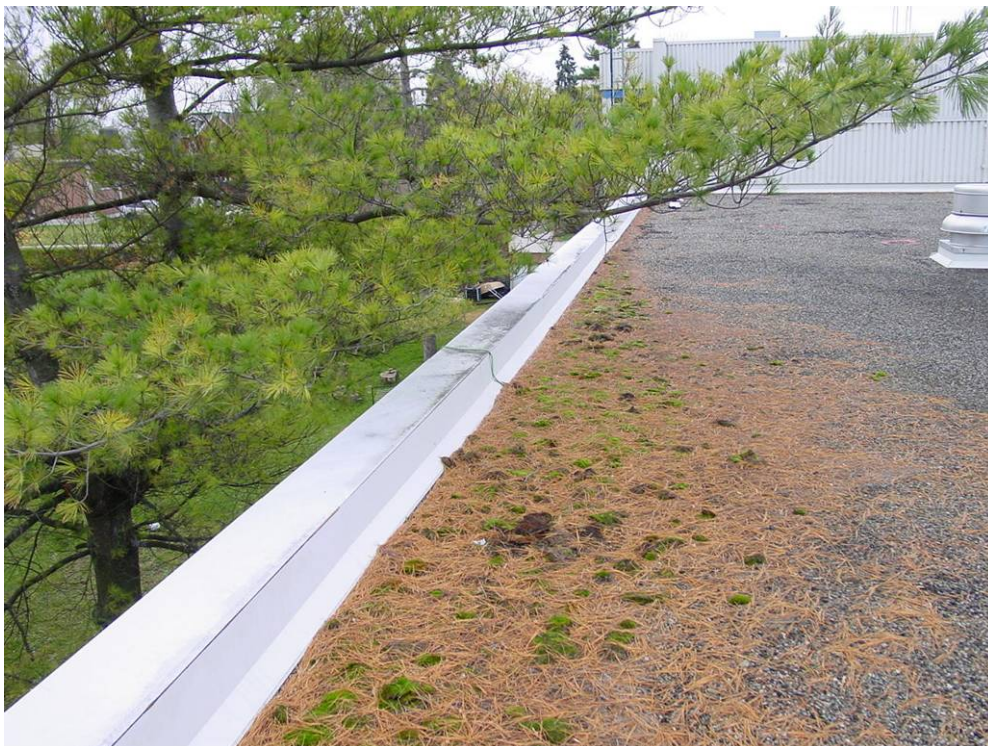
Photograph 8: Roof Area 1.1 - Heavy moss growth and organic debris exists along the south perimeter due to adjacent trees overhanging the roof. Moss is a form of vegetation that can grow on a roof surface. A roof surface with moss cover tends to deteriorate at an accelerated rate.
