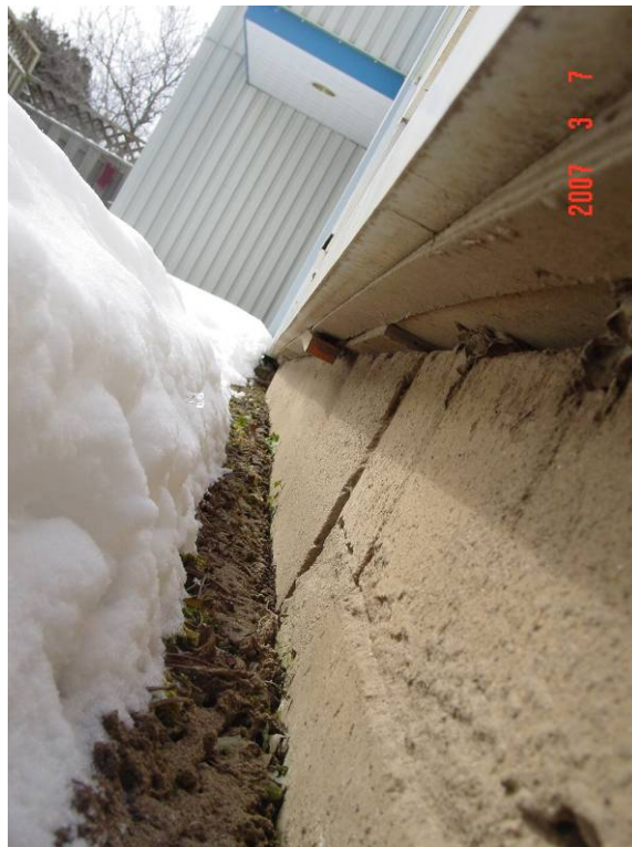
Photograph 22: At the East elevation, it was observed that no sill flashings were installed below the ground floor windows; there seemed to be plywood strips beneath, some of them being loose.
