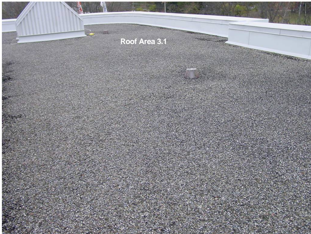
Photograph 39: Roof Area 3.1 – Overall view looking west. This roof area is situated over the Finance Department at the northwest portion of the facility. The existing roof consists of a built up bituminous membrane system installed in 1989.
