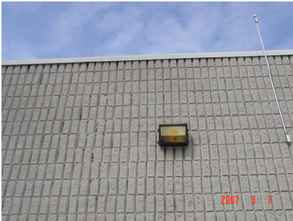
Photograph 5: The split-face concrete blocks were not aligned correctly and various mortar joints were not completely filled with mortar.
