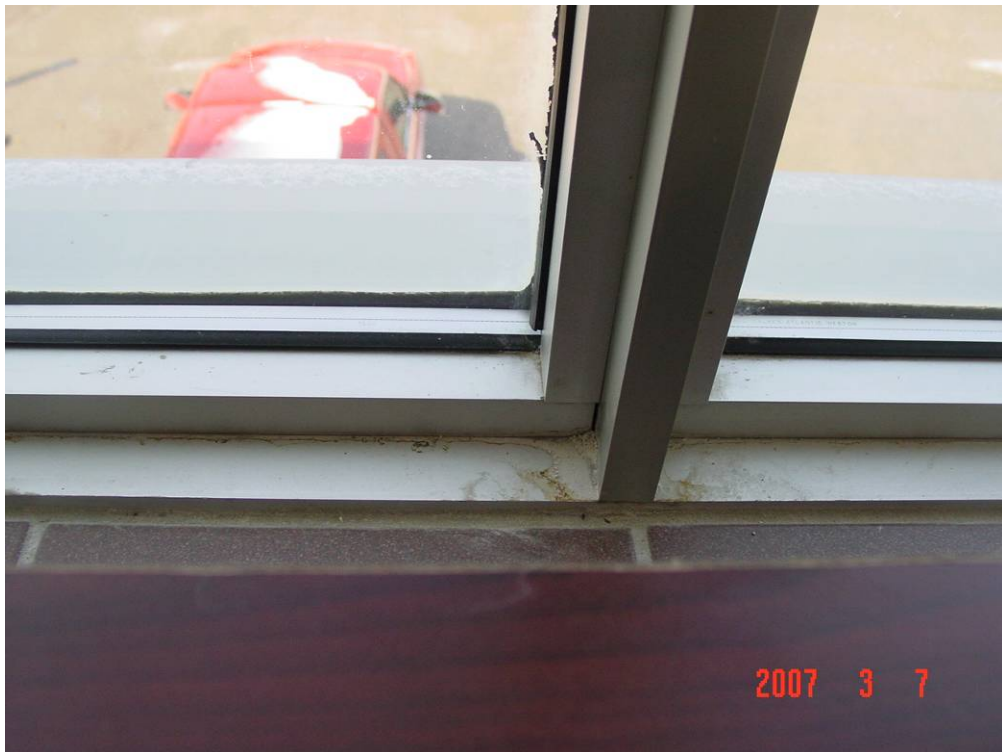
Photograph 20: Water leakage at various locations at the interior window sills/frames was evident.
