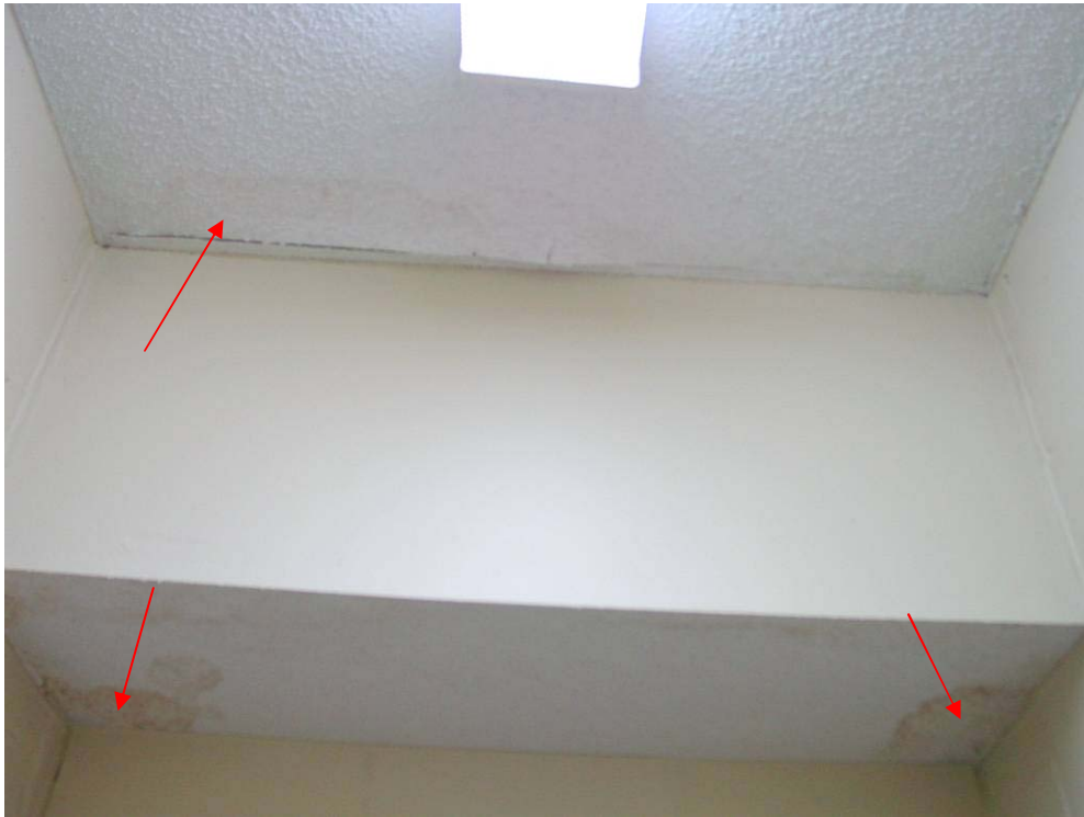
Photograph 37: Roof Area 2.2 – Interior view. Ongoing leaks were evident in the stairwell below this roof area particularly along the perimeter wall transitions.
