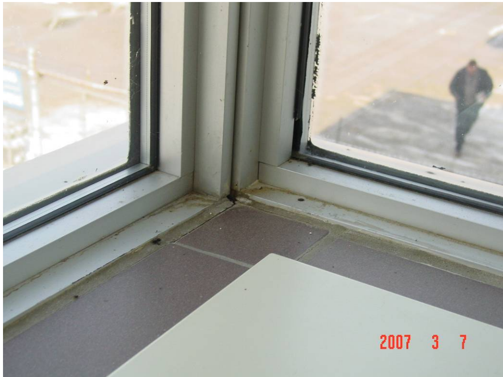
Photograph 19: Various installed glazing stops were undersized.
