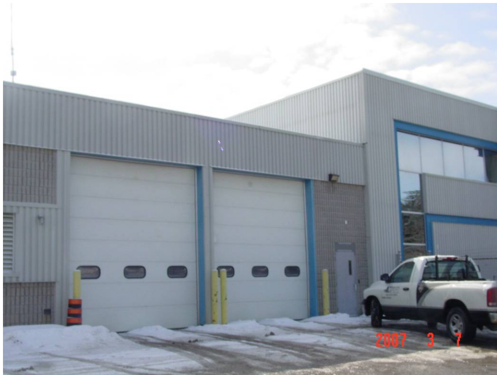
Photograph 1: Original warehouse portion of the building constructed with split-faced concrete block with siding accents to match newer addition.
