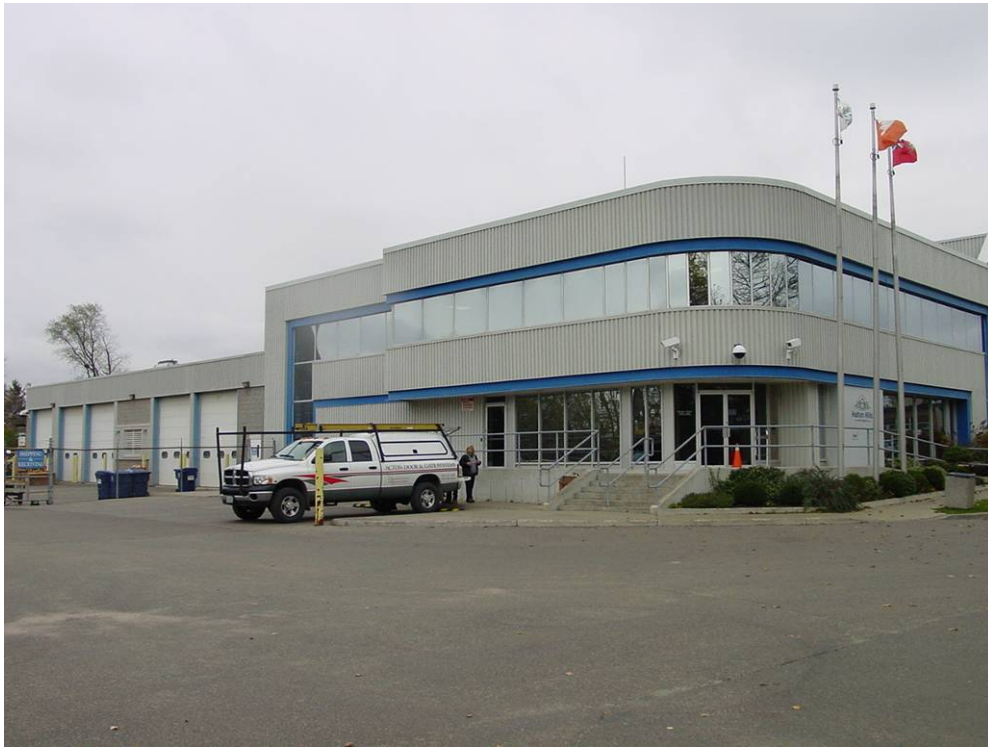
Photograph 1: Northwest elevation of the Halton Hills Hydro Building in Acton. The existing building is a multi storey steel frame and metal clad structure extensively renovated and rebuilt in 1989.
