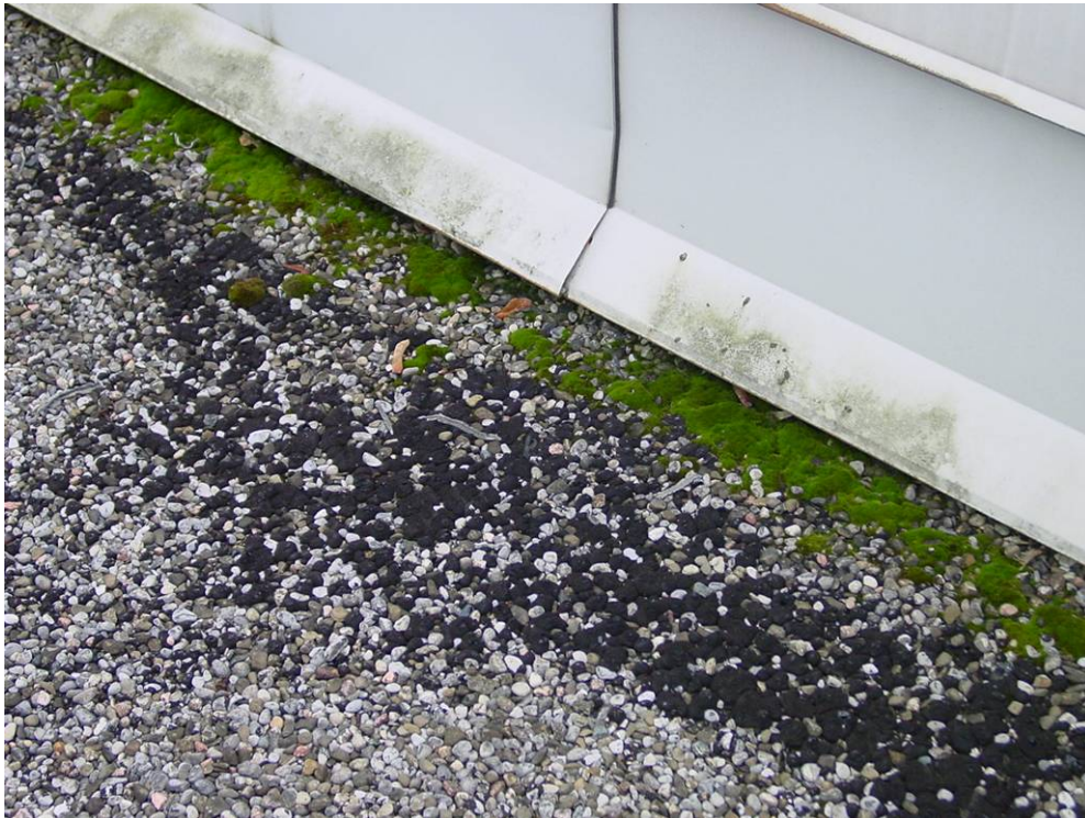
Photograph 43: Roof Area 3.1 - Localized moss growth exists at corner transitions and along the base of the south skylight.
