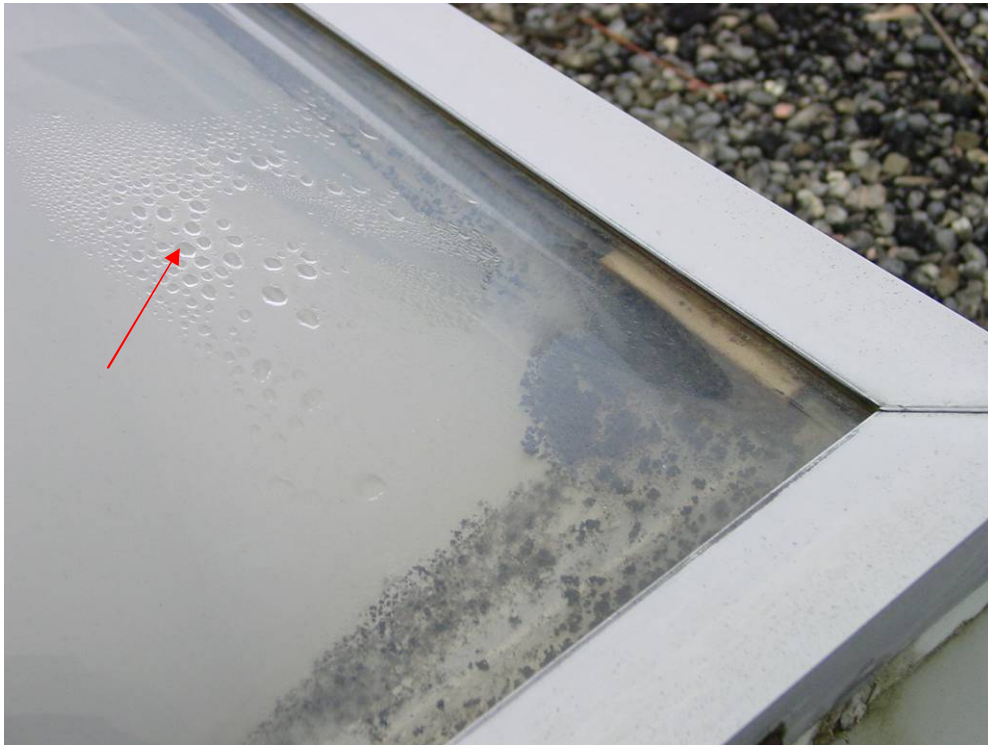
Photograph 35: Roof Area 2.1 – There is evidence of long-term moisture accumulation between the panes of the skylights and it is likely that the seal between the panes has failed. This condition may be contributing to the reported water entry into the space below.
