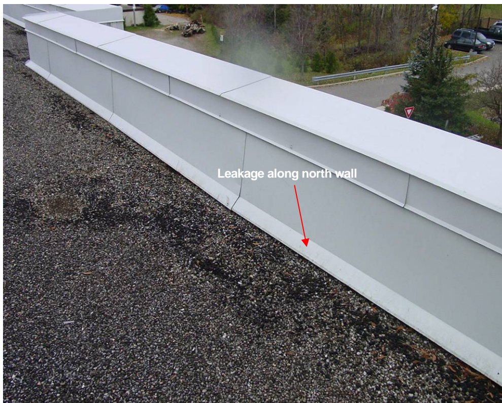
Photograph 46: Roof Area 3.1 – Photo of the north parapet in the vicinity of the leaks above Manager of Engineering office.
