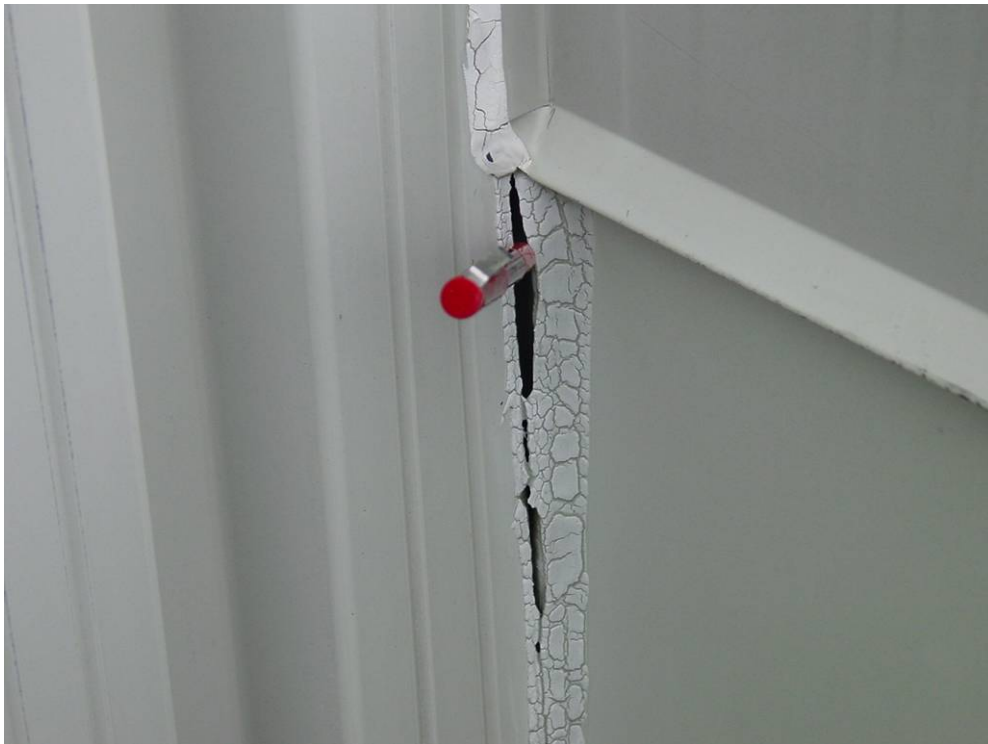
Photograph 32: Roof Area 2.1 – Sealant deterioration exists at the metal flashing and cladding joints in the northwest corner. Reported leaks below this location (see photo 31 above) could be due to wind blown moisture entering through the failed sealant.
