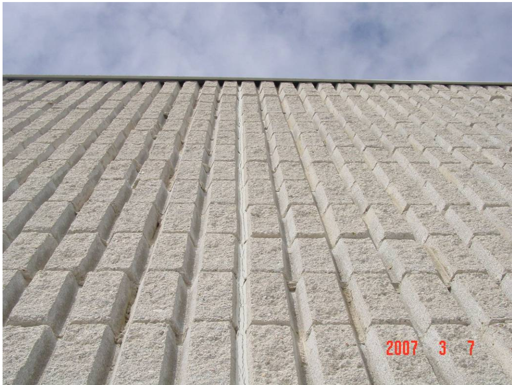
Photograph 3: In general, the exterior masonry walls are in good to fair condition with very minor deterioration observed.
