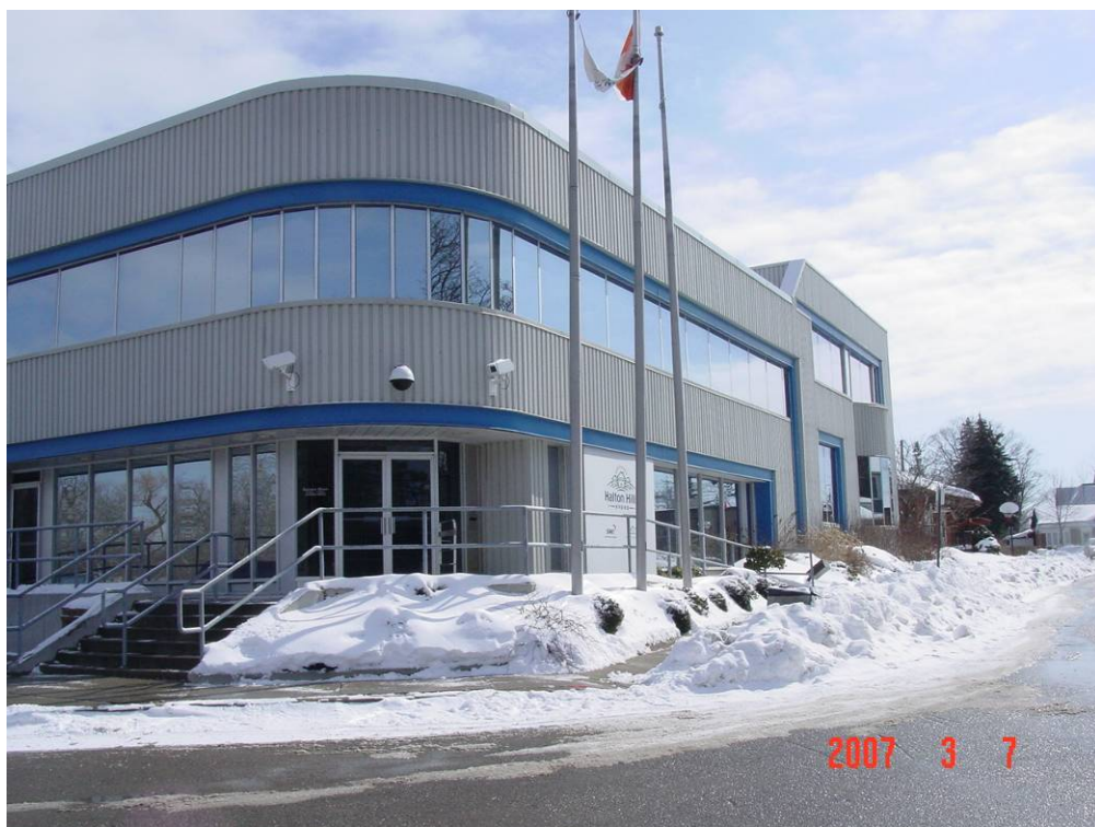
Photograph 2: The addition is a steel structure with prefinished steel siding supported on concrete footings with concrete block foundation walls.
