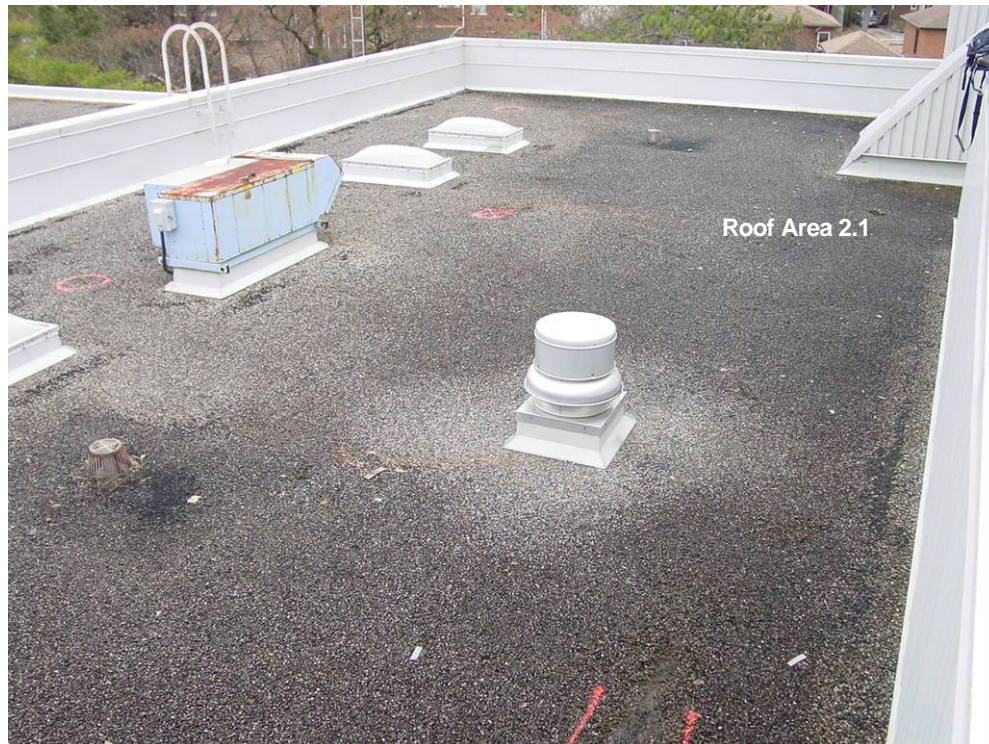
Photograph 21: Roof Area 2.1 - Overall view looking south at roof area 2.1 situated over the Engineering Department in the central portion of the building. The existing roof consists of a built up bituminous membrane system installed in 1989.
