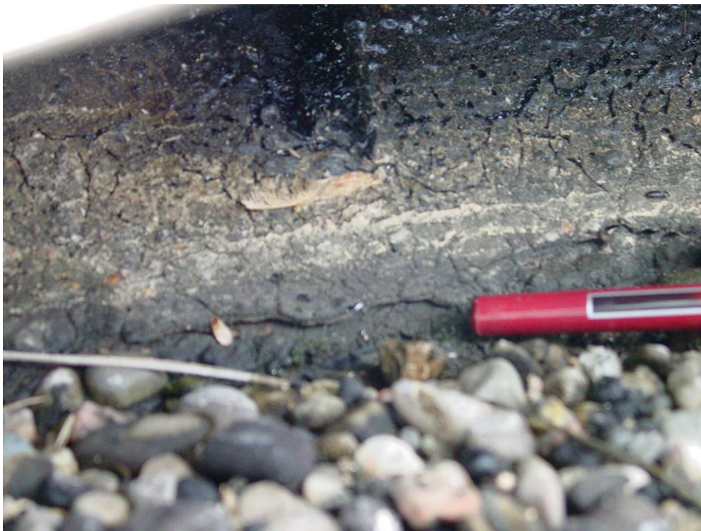
Photograph 28: Roof Area 2.1 – Existing membrane flashings at perimeter parapets and curb penetrations are exhibiting developing deterioration and exposure (photograph 15). Cracking of the membrane flashings along the base of the north wall is a potential source of the reported leaks over the north end of the Engineering Department.
