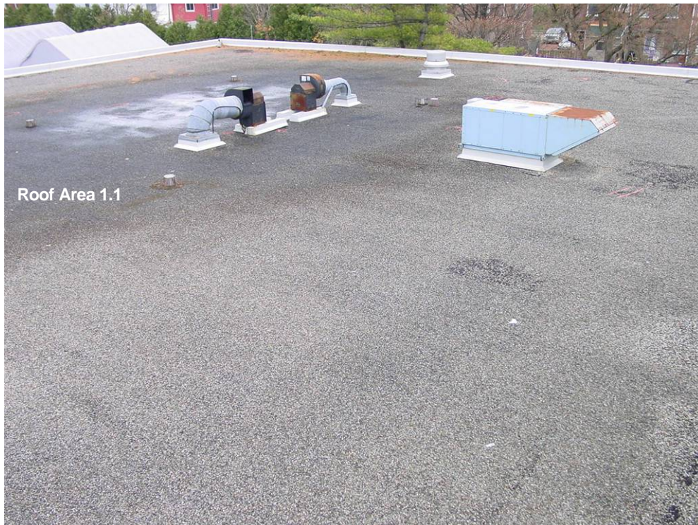
Photograph 3: Roof Area 1.1 – Overall view looking northeast at roof area 1.1 situated over the Garage in the east end of the facility. The existing roof consists of a built up bituminous membrane system installed in 1989.
