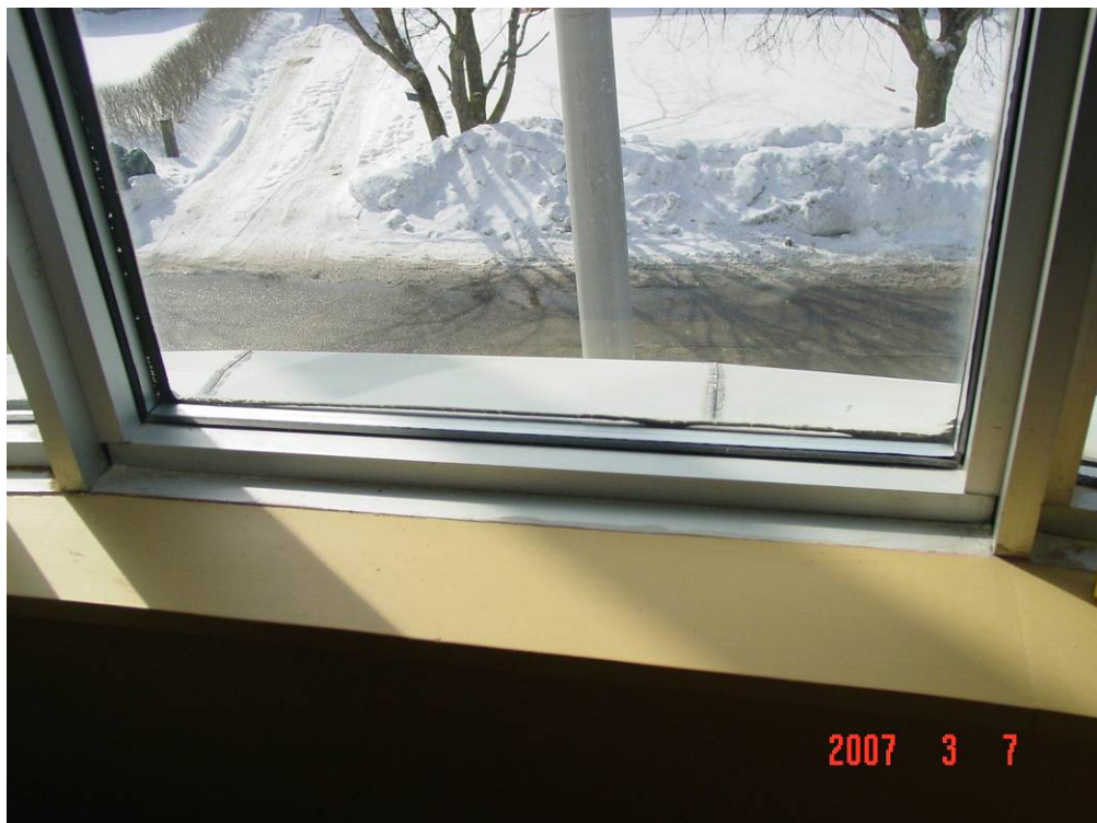
Photograph 18: Aluminum sills have been provided at the base of the 2 nd floor windows. This was observed from the interior of the building.
