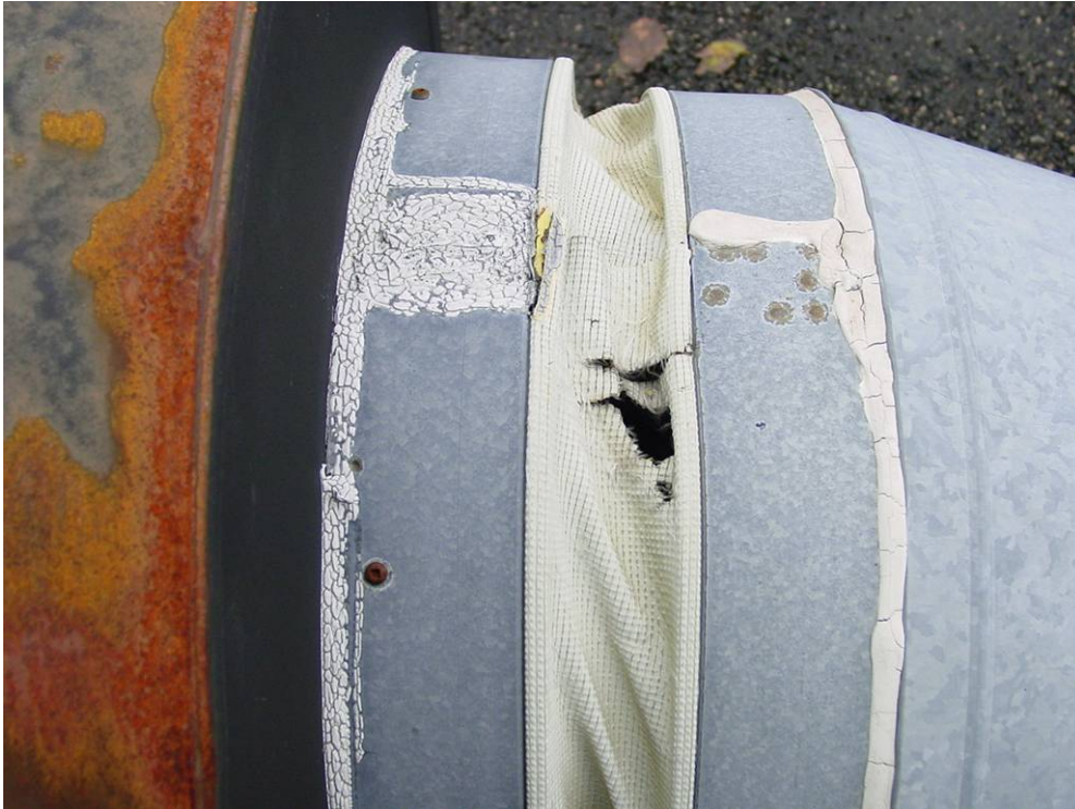
Photograph 15: Roof Area 1.1 – Water entry is likely at the deteriorated flexible duct connections.
