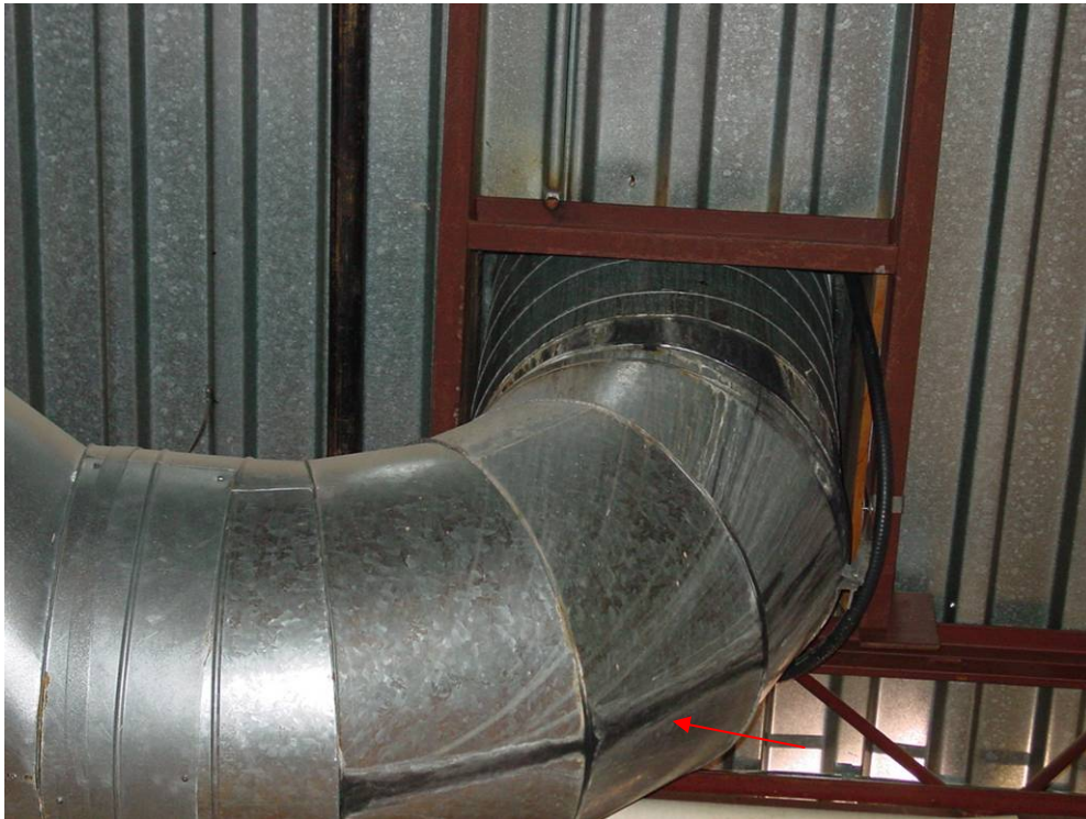
Photograph 13: Roof Area 1.1 – Ongoing leaks were reported below the north exhaust duct opening. Water stains are evident around spiral duct.
