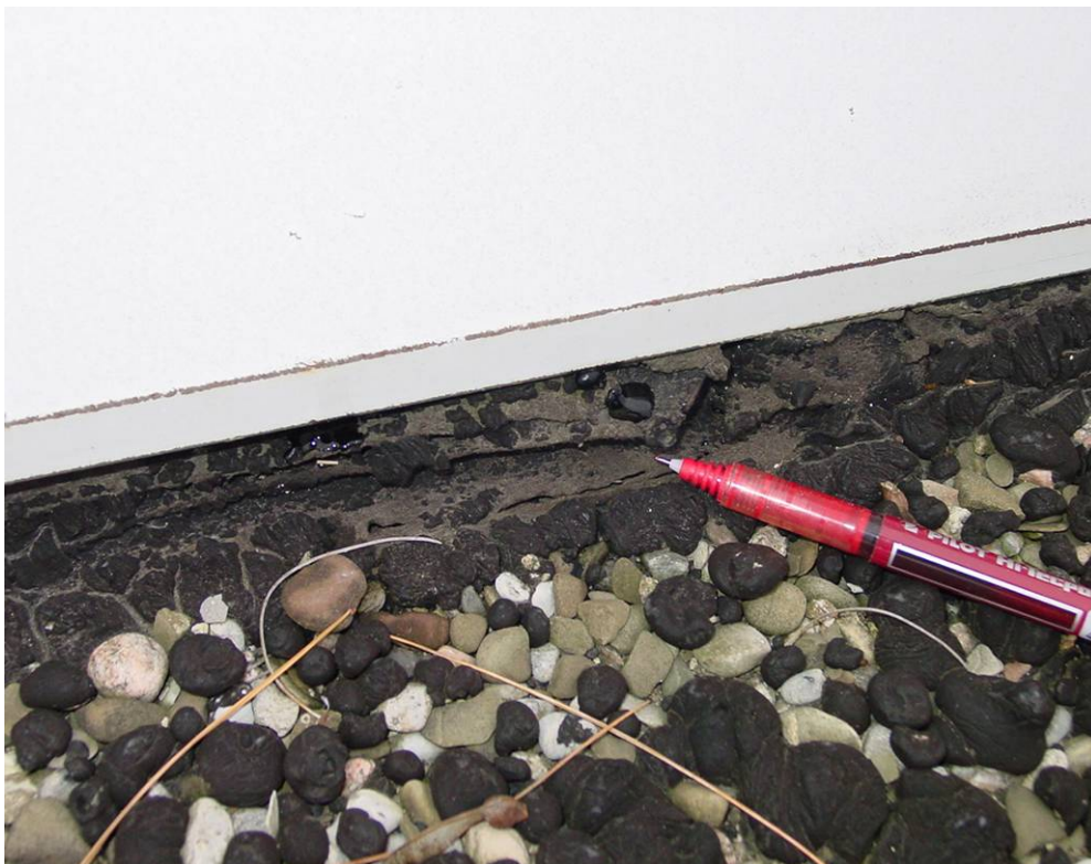
Photograph 10: Roof Area 1.1 - Existing membrane flashings at perimeter parapets are exhibiting developing deterioration, delamination and embrittlement.
