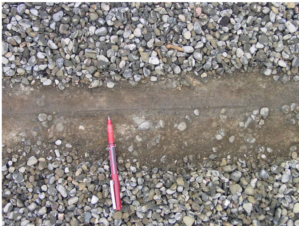
Photograph 42: Roof Area 3.1 – Photo showing evidence of poor floodcoat coverage and adhesion. This condition leads to premature wear and deterioration of the top membrane plies.
