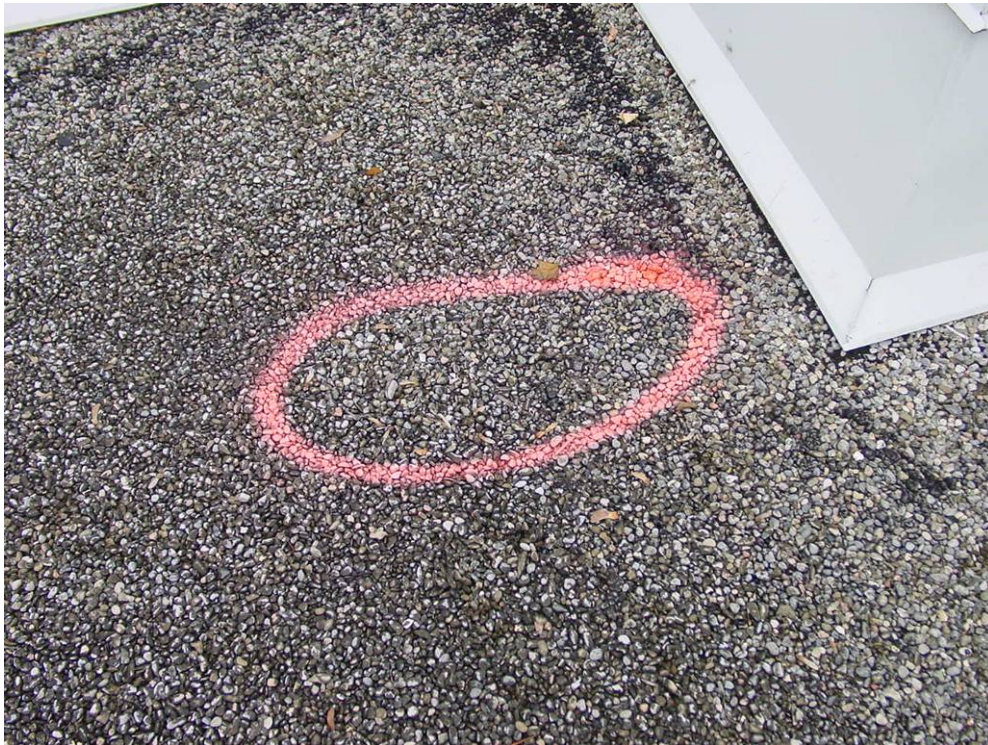
Photograph 53: Roof Area 4.1– Localized membrane blistering is evident.
