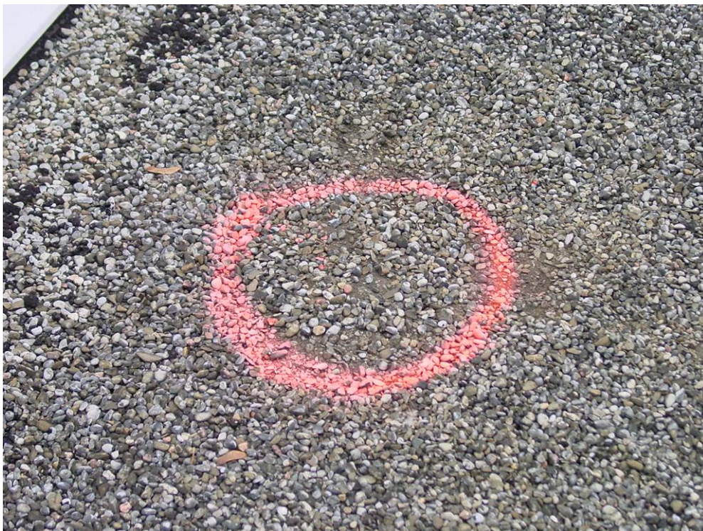
Photograph 44: Roof Area 3.1 – Localized membrane blistering is evident.
