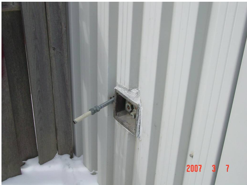
Photograph 12: Sealant deterioration at wall penetrations.
