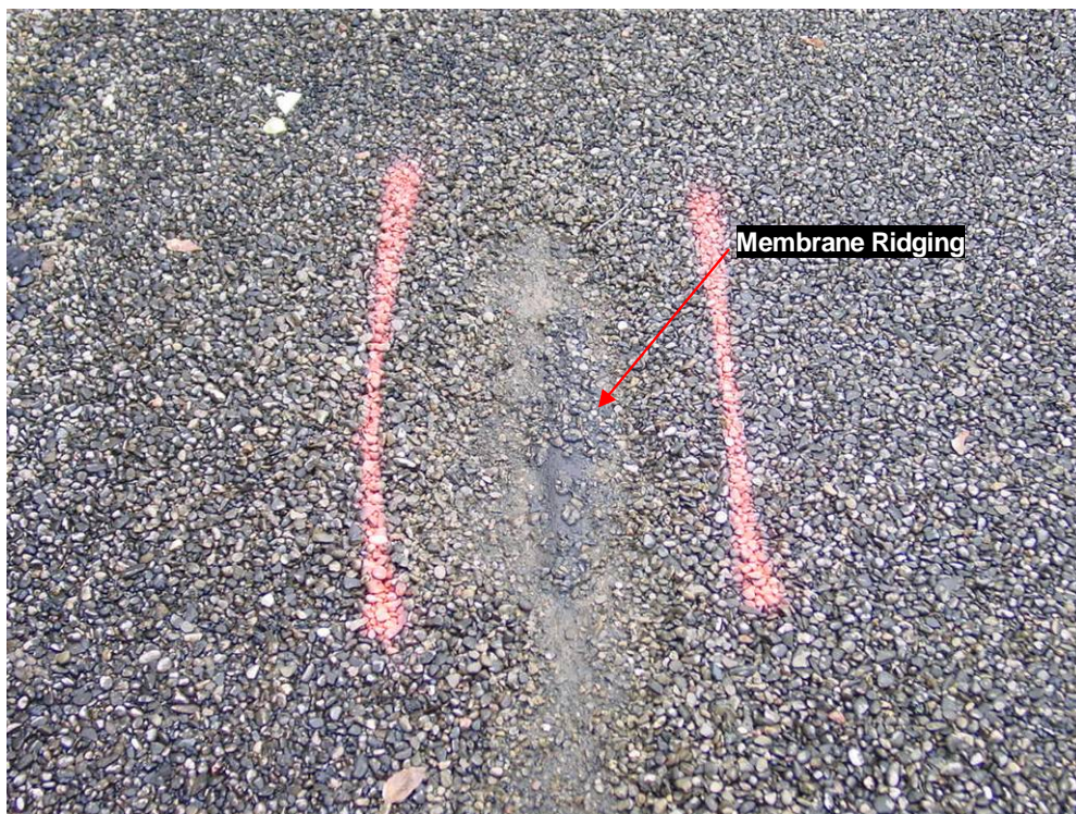
Photograph 26: Roof Area 2.1 – Localized membrane ridging and blistering was evident throughout the roof area.
