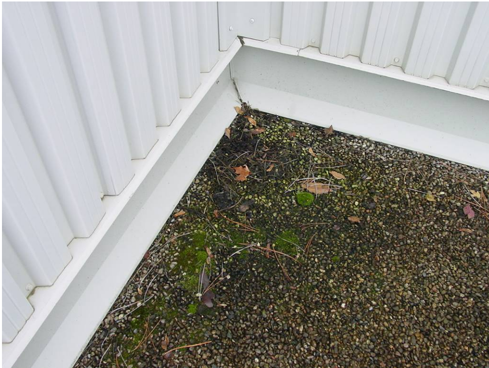
Photograph 29: Roof Area 2.1 – Localized moss growth and organic debris exists at corner transitions.
