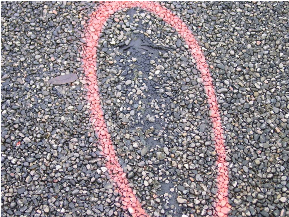
Photograph 9: Roof Area 1.1 – Heavy membrane blistering and ridging is evident in localized areas throughout the roof.
