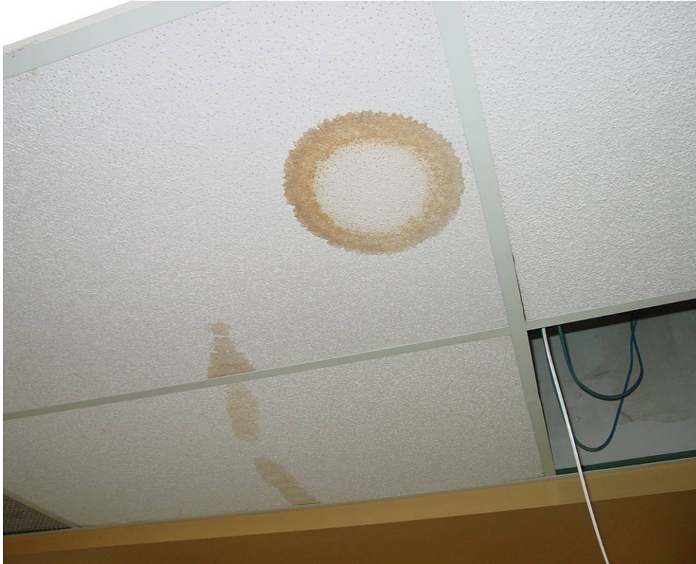
Photograph 31: Roof Area 2.1 – Water stained ceiling tile was noted over workstation in northeast corner.
