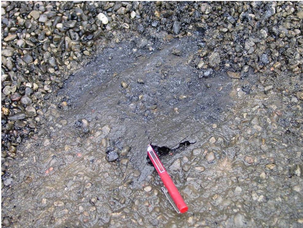
Photograph 27: Roof Area 2.1 – A broken blister was evident in the northwest corner and may be a source of leakage.
