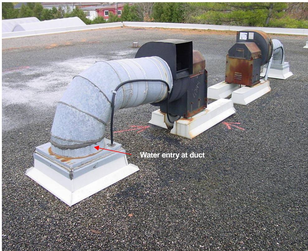
Photograph 14: Roof Area 1.1 – Photograph showing the duct penetrations (area of leaks) above the garage.
