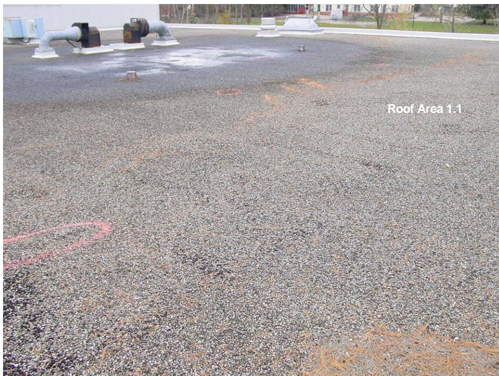
Photograph 4: Roof Area 1.1 – Overall view of roof area 1.1 looking northwest. Drainage patterns appear to be generally good due to a slightly sloping structural substrate.
