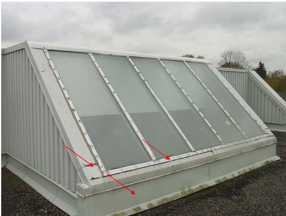
Photograph 48: Roof Area 3.1 – A history of leaking was reported along the base of the south skylight.
