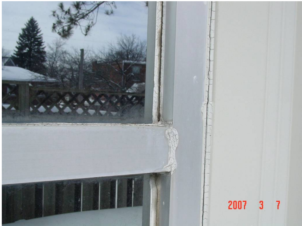
Photograph 11: Sealant deterioration at the window perimeters.
