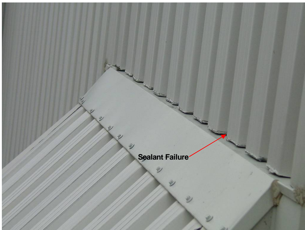
Photograph 38: Roof Area 2.2 – Investigation revealed that sealant failure along the upper west wall transition is a possible source of water entry. If inadequate membrane waterproofing was installed under the metal panels, then any water entering through failed sealant could more readily enter the building.
