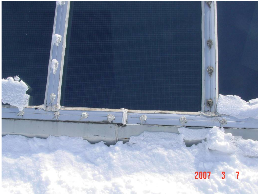
Photograph 15: Improper overbeading repairs to the sealant joints at the skylights.
