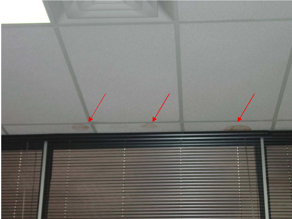
Photograph 45: Roof Area 3.1 – Water stained ceiling tile was observed along north wall of Manager of Engineering office.
