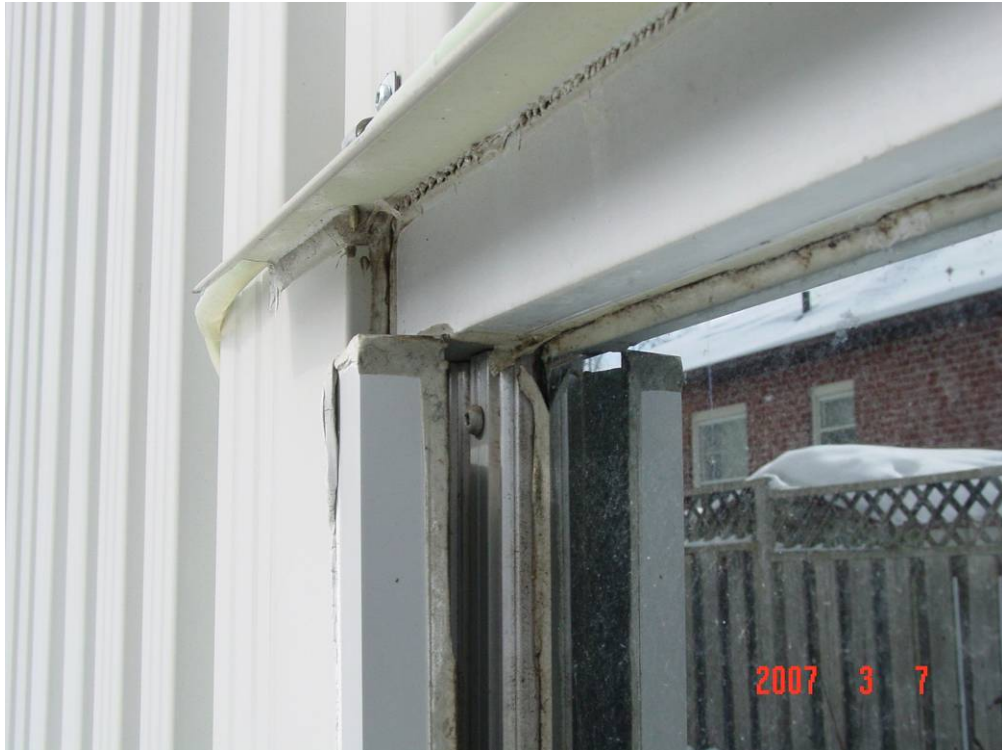
Photograph 23: Some glazing cover caps were noted to be loose.
