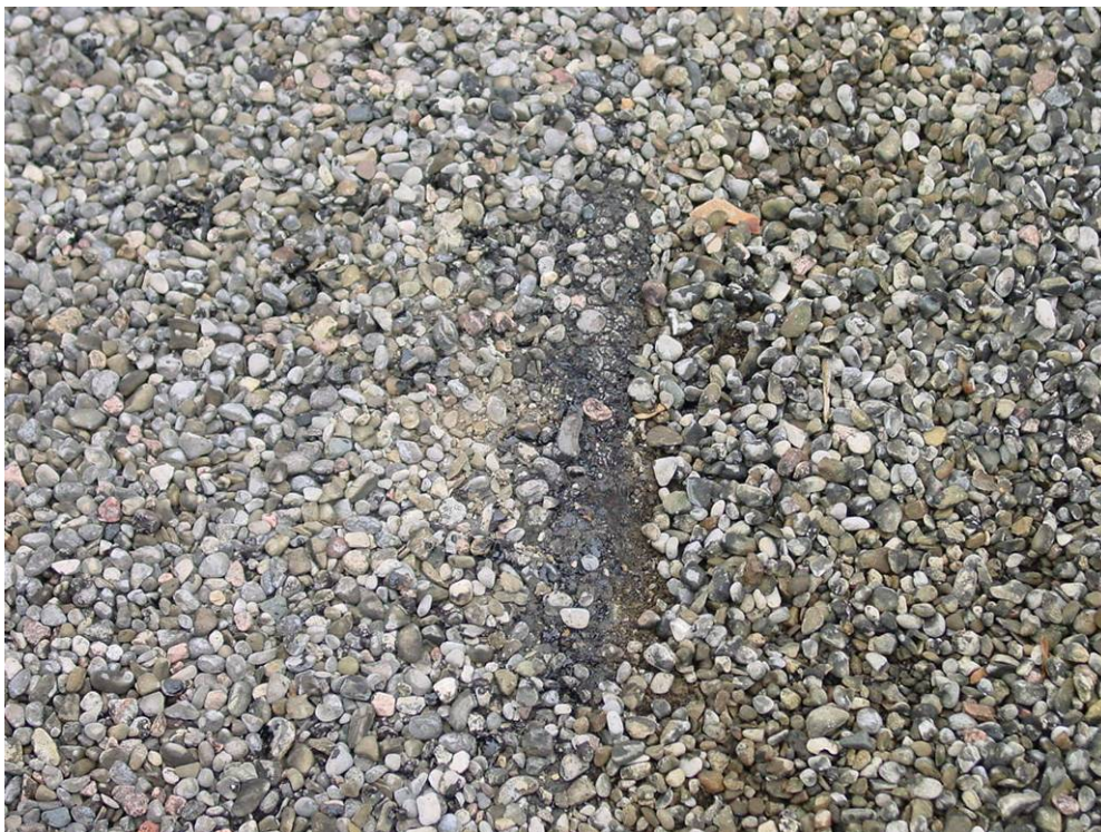
Photograph 54: Roof Area 4.1- Membrane exposure was identified along the transition between roof area 4.1 and 4.2.
