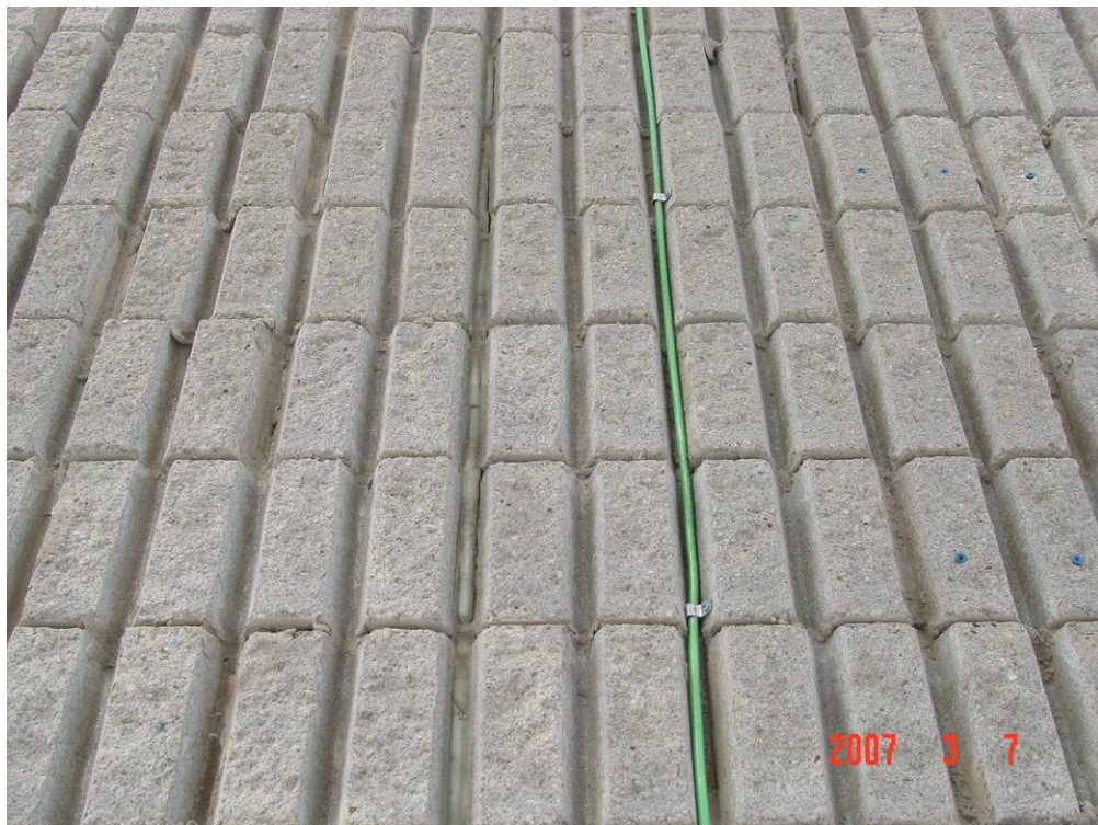
Photograph 10: Sealant deterioration at the control joints at the full height of the concrete block walls.
