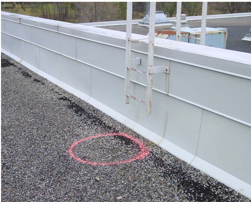
Photograph 30: Roof Area 2.1 – No membrane protection has been provided at the base of access ladders. Membrane blistering and delamination was evident at the base of the east roof ladder. Active roof leaks were reported below the ladder along the east parapet shown above.
