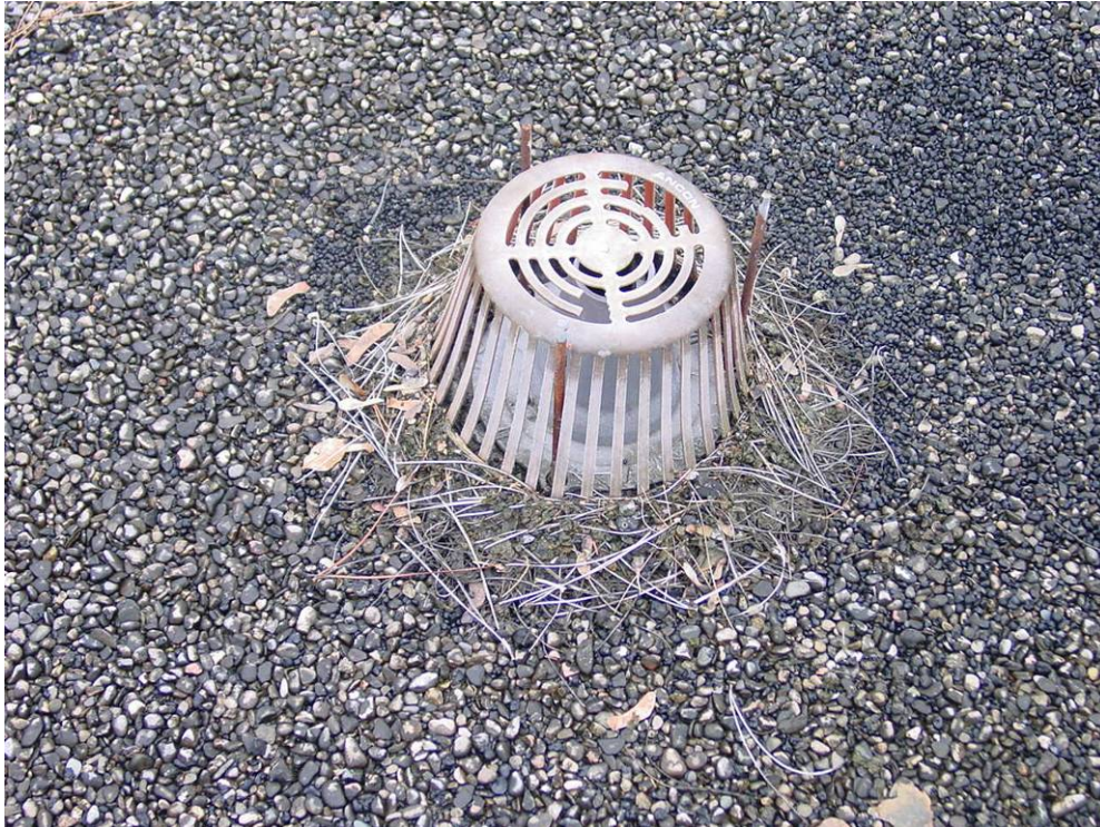
Photograph 25: Roof Area 2.1 – Drainage patterns appear to be generally good with evidence of ponding due to debris accumulation around drains.
