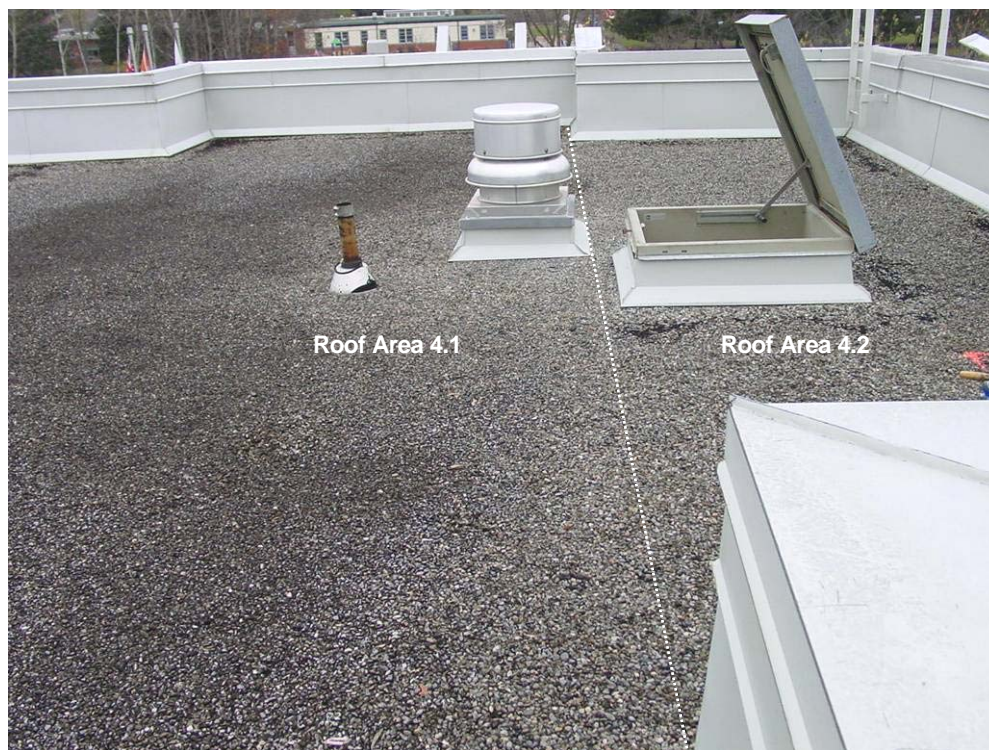
Photograph 50: Roof Areas 4.1 and 4.2 – These uppermost roof areas are situated over the southwest corner of the building and consist of built up bituminous membrane systems installed in 1989.
