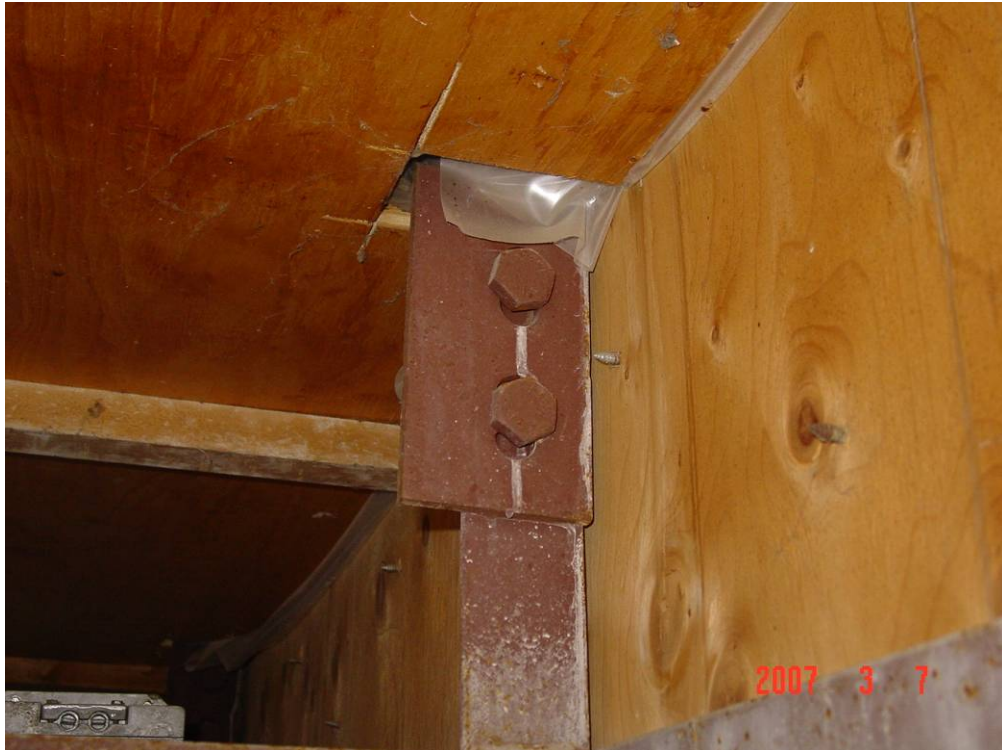
Photograph 27: At soffit locations where the plywood was cut out around the structural steel framing, it did not appear that the polyethylene air/vapour barrier was sealed.
