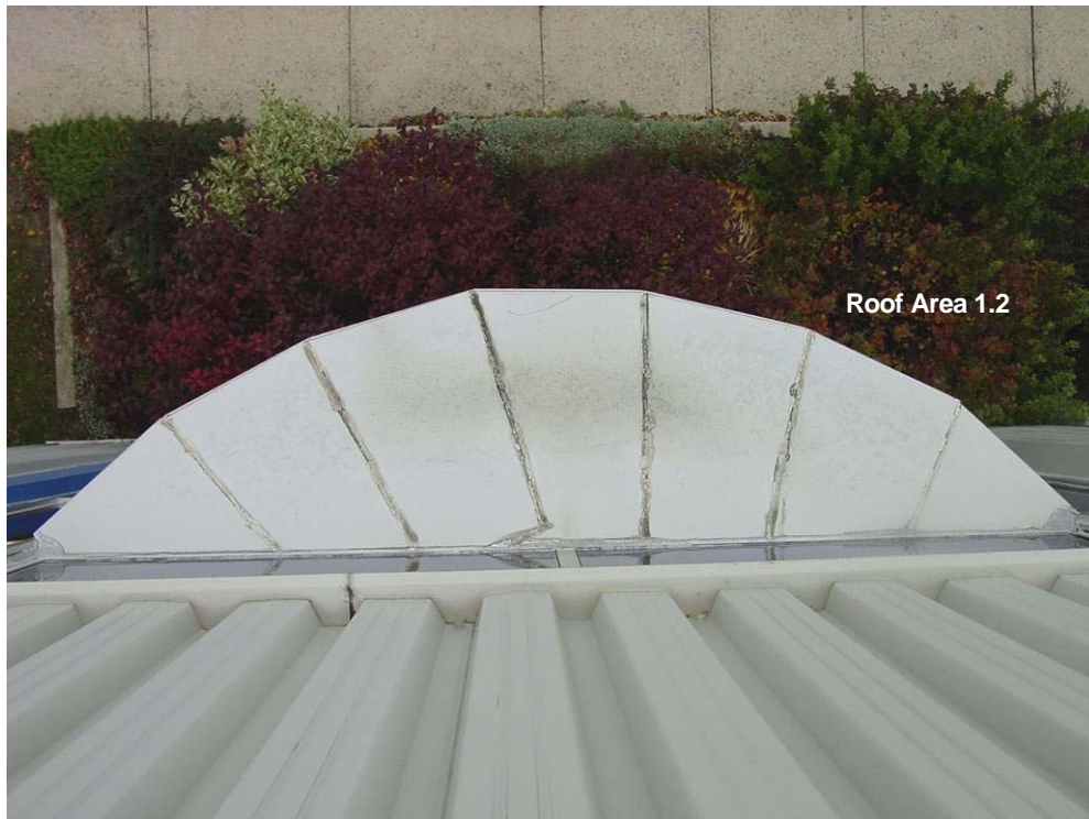
Photograph 19: Roof Area 1.2 - This small roof area is situated over the lunchroom bay window along the west perimeter of the building. The existing roof consists of prepainted metal panels, installed in 1989.
