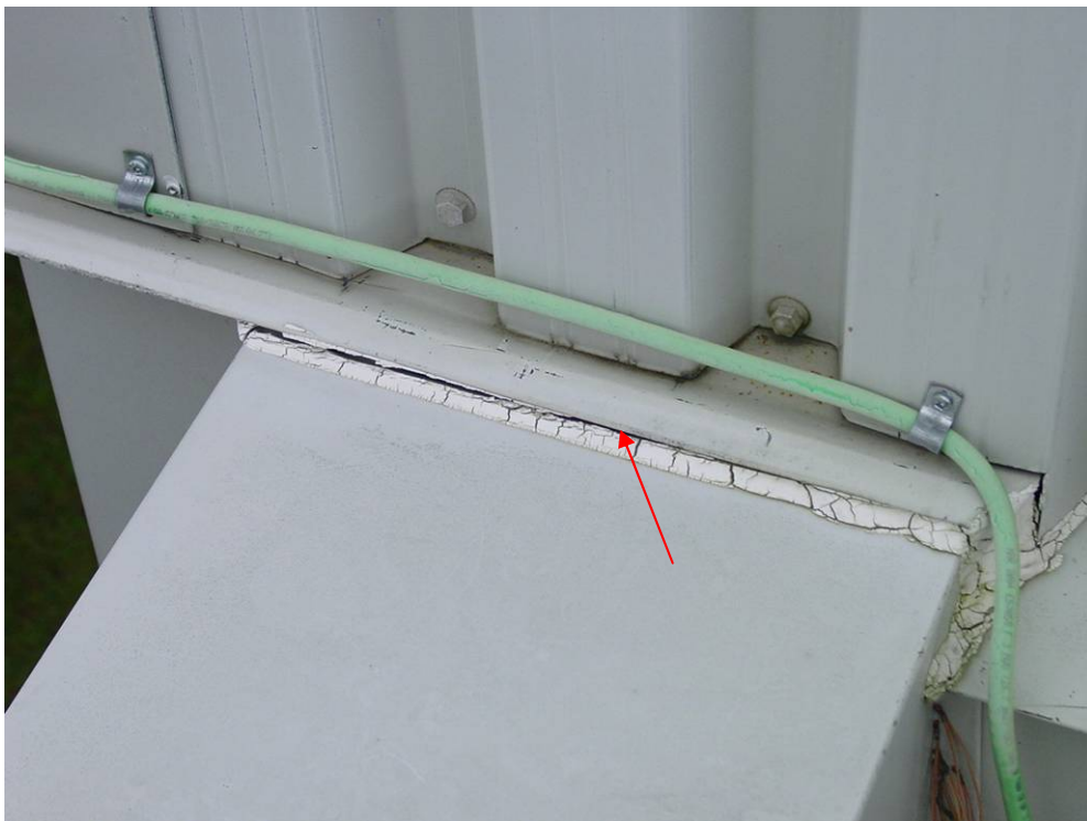
Photograph 12: Roof Area 1.1 - Sealant deterioration exists at metal flashing joints and transitions, adding to the potential for wind blown moisture to enter the building.
