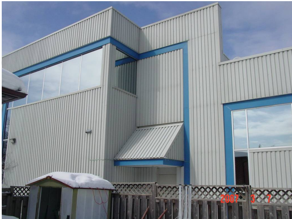
Photograph 7: The exterior prefinished steel siding was generally in good condition.
