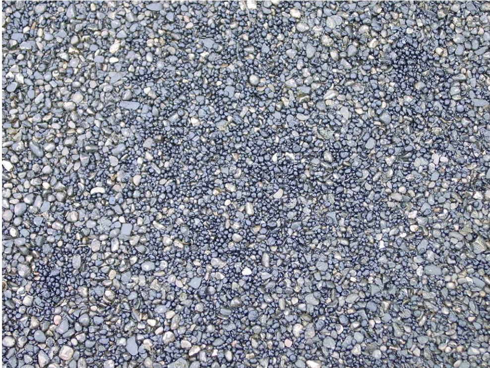
Photograph 7: Roof Area 1.1 – Generally heavy bitumen bleedthrough and blueberry accumulation was noted throughout the area. These anomalies are associated with weathering and aging of the roof system.
