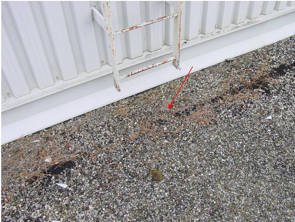
Photograph 11: Roof Area 1.1 – No membrane protection has been provided at the base of the access ladder along the west wall. The membrane at this area typically experiences additional stress and potential damage from foot traffic, impact loading and erosive forces. Walkway pads or concrete pavers are appropriate elements for such areas.
