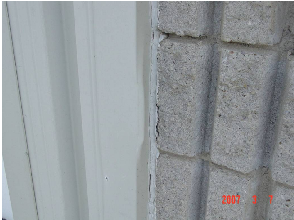
Photograph 9: All observed sealant joints at all elevations were in very poor condition, which included all sealant joints between the siding and the split-faced concrete block.
