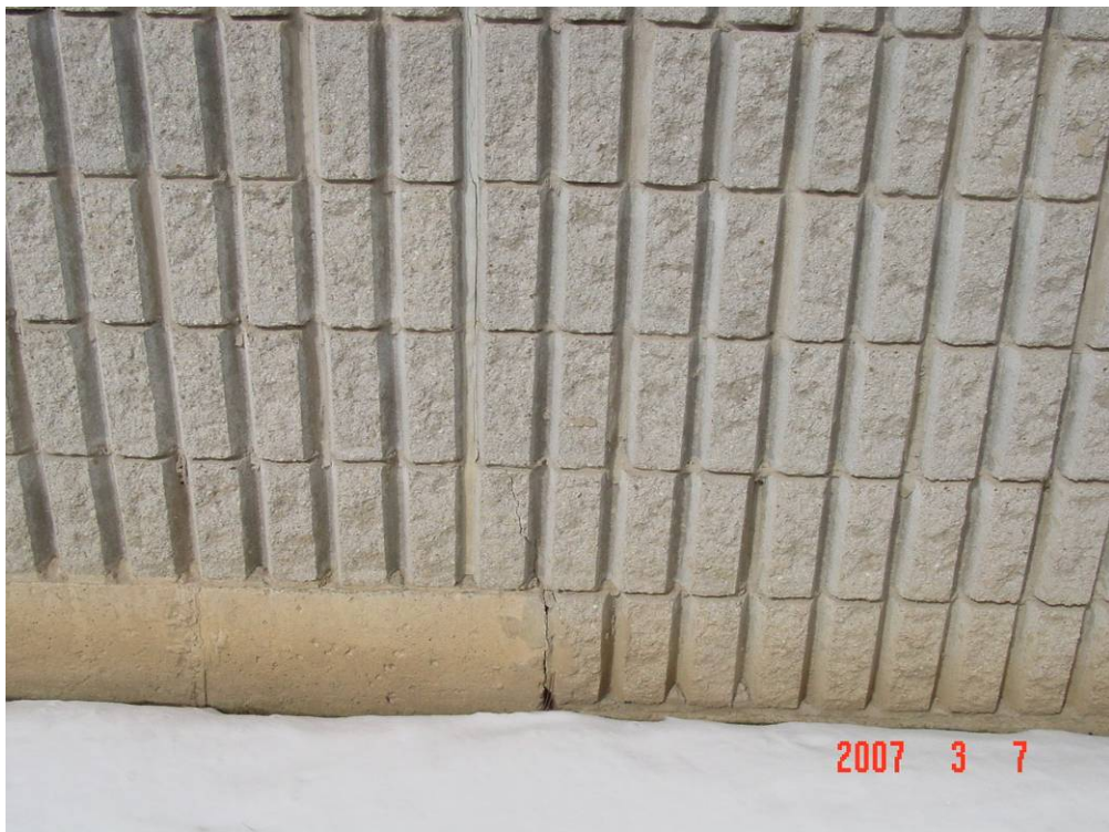
Photograph 6: Cracked concrete blocks were only visible at one (1) location, above a stepped foundation wall at the East elevation.
