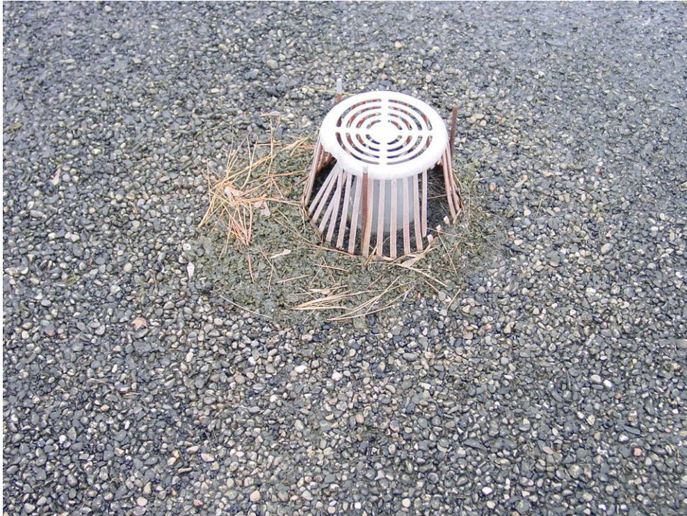
Photograph 5: Roof Area 1.1 – Localized ponding is evident along the central portion of the roof area primarily due to debris obstructing the roof drains.
