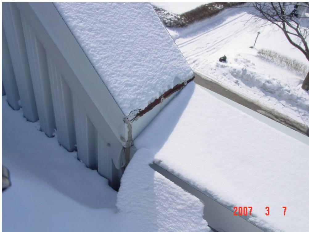
Photograph 8: The metal parapet cap flashings were in very good condition as well except at one (1) location, at the sloped parapet at the South elevation.
