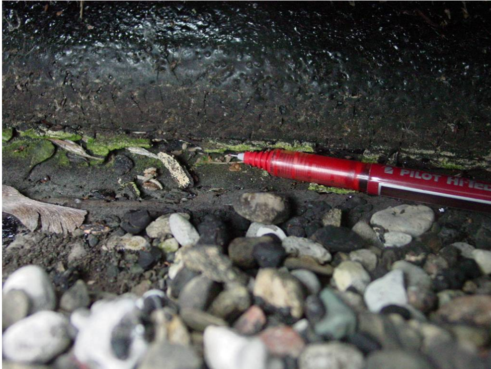
Photograph 47: Roof Area 3.1 North Wall – Investigation revealed splits in membrane flashing above the leak location.
