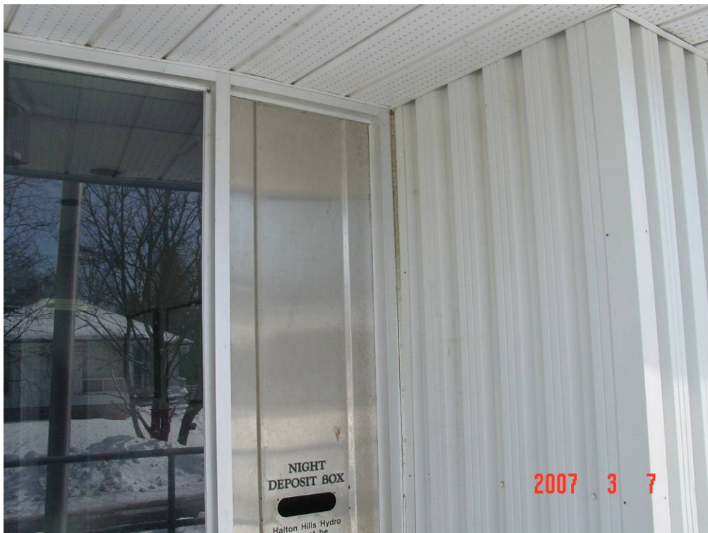
Photograph 24: Within the vestibule, Halton Hills Hydro has installed a 'Night Deposit Box', a steel panel en lieu of the window at this location. The steel panel is not insulated and there are obvious holes at the corners of the window frame
