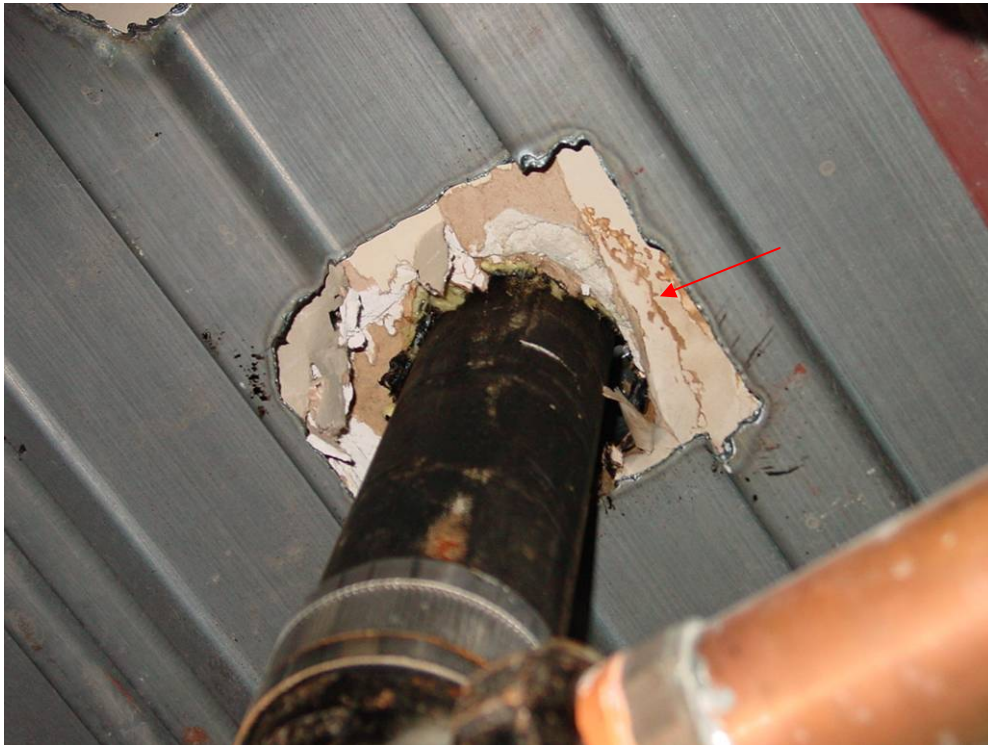
Photograph 33: Roof Area 2.1 – Water stained drywall was noted at a leak location above the corridor leading to the payroll department.
