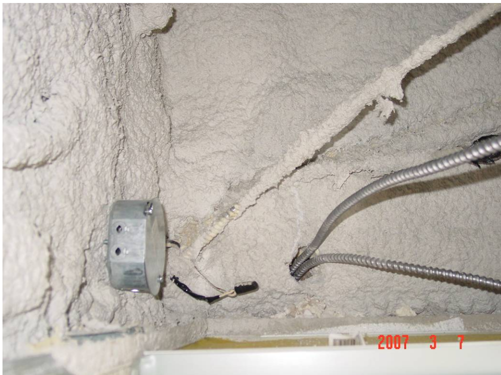
Photograph 28: At one location between the soffit and the main floor ceiling space, an opening in the polyurethane foam was noted at an electrical conduit.
