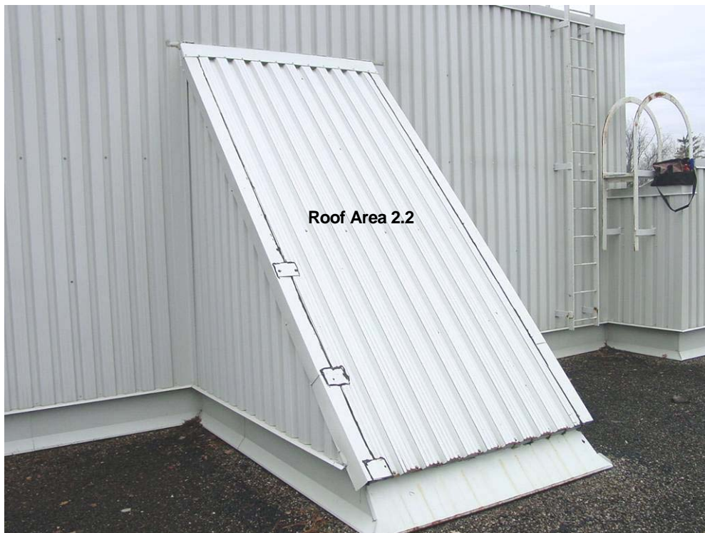
Photograph 36: Roof Area 2.2 – This small roof area is situated over the stairwell leading from the second floor level to the Engineering Department at the southeast portion of the building. The existing roof consists of prepainted metal panels installed in 1989.
