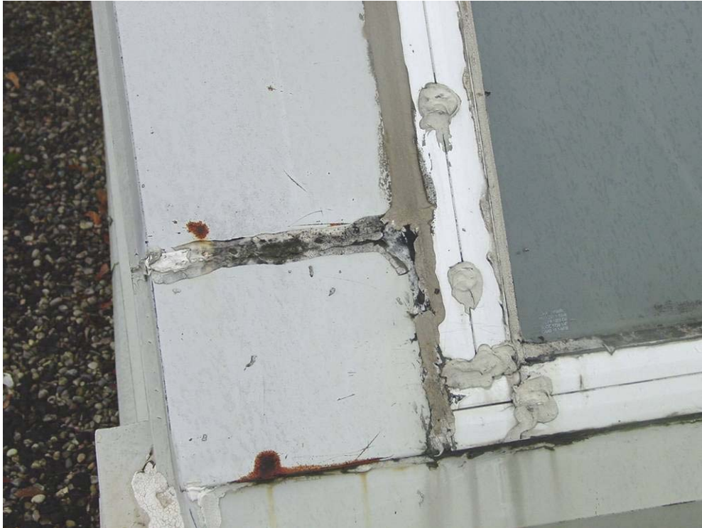
Photograph 49: Roof Area 3.1 - Visual review of this skylight indicated that sealant deterioration could be resulting in water entry. In addition, deterioration of the membrane flashings along the base of the skylight could be contributing to the water entry. Previous caulking repairs were evident throughout the skylight.
