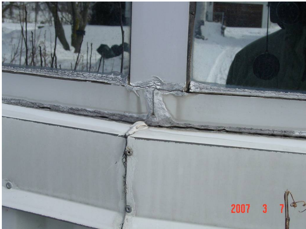
Photograph 14: Sealant deterioration at all glass-to-metal sealant joints.
