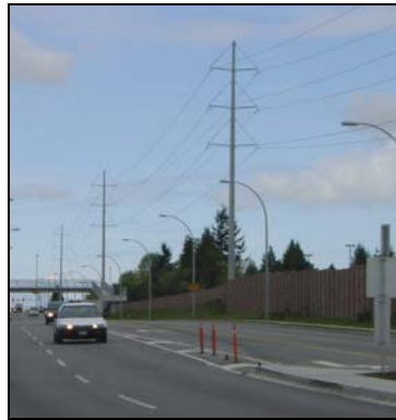
230kV Double Cct Mono-tube Steel Pole (Right Side of Photo) – Vertical Conductor Spacing
