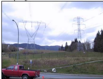
230kV Double Cct Mono-tube Steel Pole (Right Side of Photo) – Vertical Conductor Spacing
