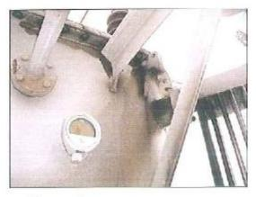
Membrane on explosion vent of station transformer damaged.
