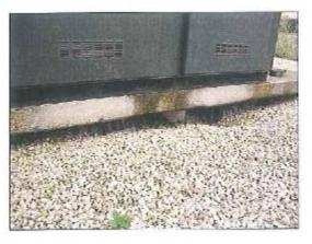
Warning sign for de-engerized operation of primary fuses not legible. OESC 36-006 (3)
