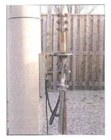
No interlock on Air break switch OESC 36-006 (2)
