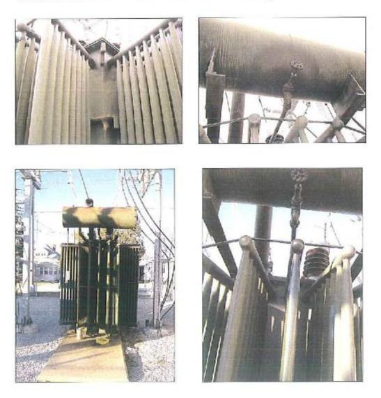
· Paint on station transformer faded
