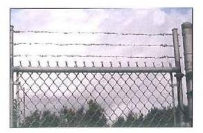
Not enough gravel in station, too large of a gap at bottom of fence fabric. OESC 26-312 (3)
