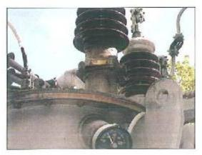
Chip out of II2 bushing on station transformer. Appears to have been painted already. Not clear on type of treatment used for repair.
