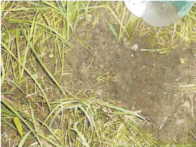
Plate 3 Close-up of Test Pit in Progress on the South Side of Victoria Street East
