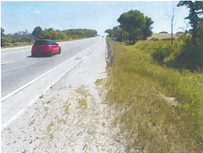
Plate 9 Highway 89, View East of South Side
