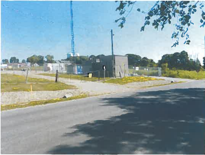
Plate 1 Cookstown Gate Station, View Northeast
