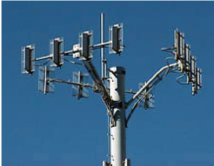
Picture of a 3 sector site.
