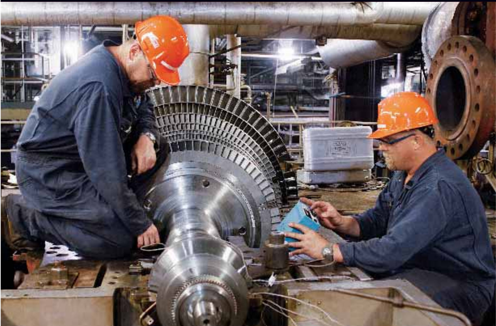
OPG employees retrofit a new boiler feed pump at the Lambton fossil-fuelled station
