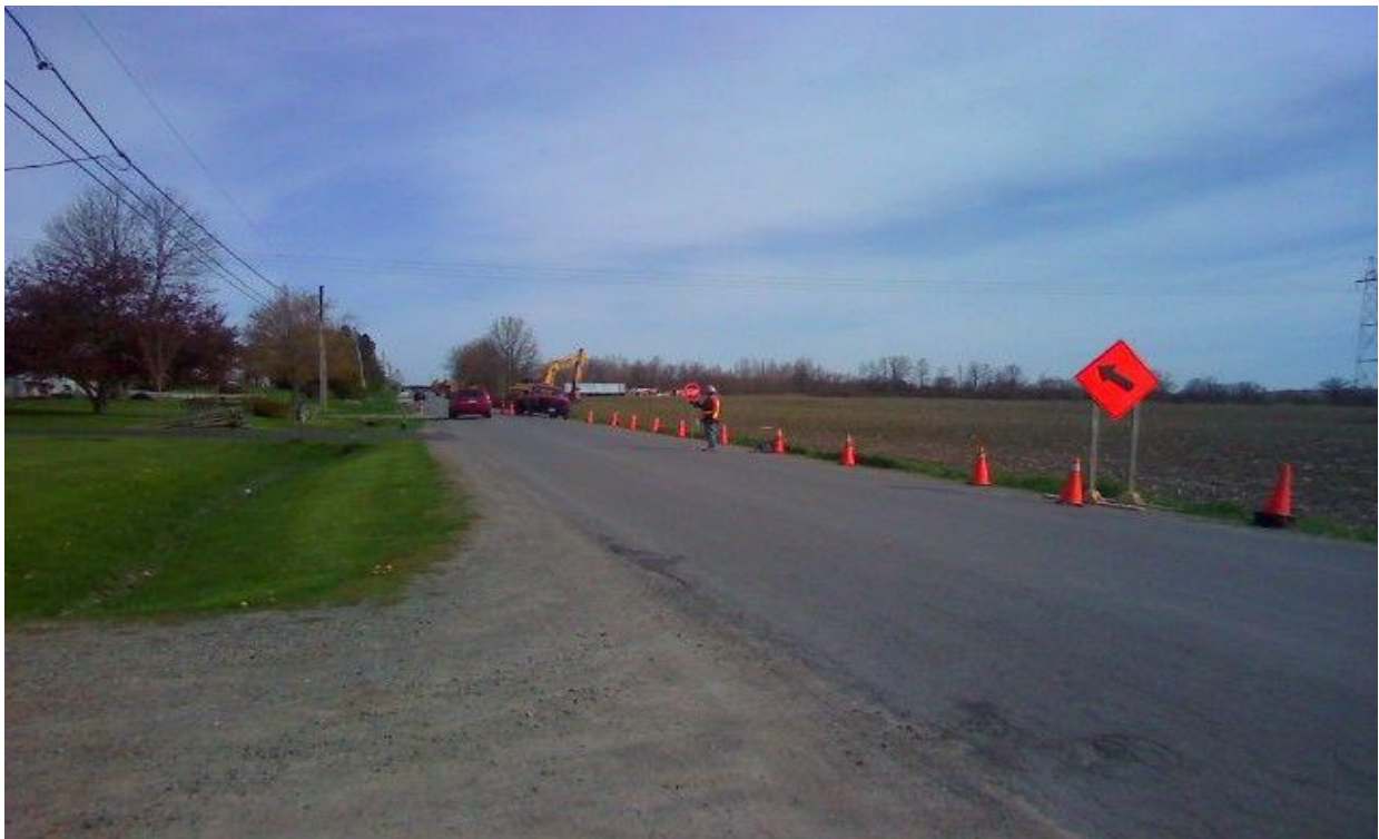
When necessary traffic was limited to one lane. Proper signage and flag persons were used to control traffic flow during these periods.
