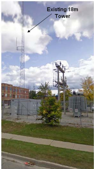
MS431 - Alliston (Replace existing 18m Tower with new 29.26m WiMax Tower)
