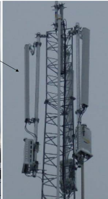
3-Sector WiMax Base Station (Base Station + Antenna's)
