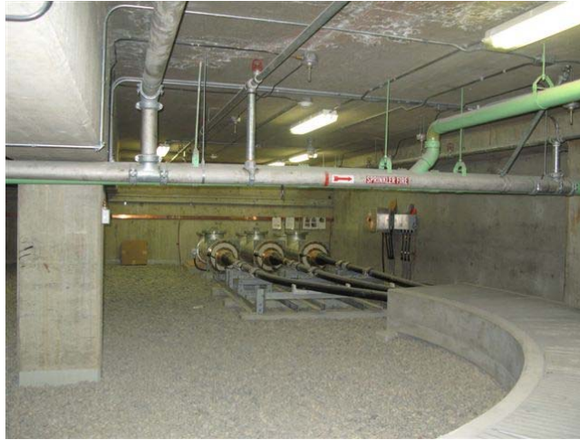
Photo 4 – Incoming 230 kV Cables for 3 rd Transformer at Interstitial Level
