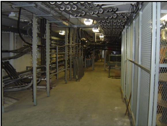
Figure 3: Windsor Station Cable Congestion
