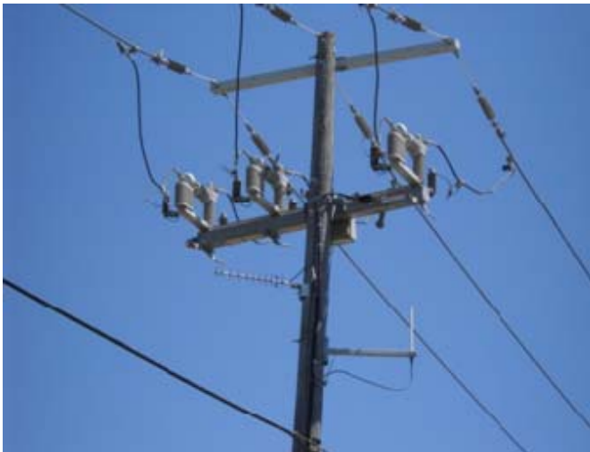
Figure 1: SCADA Switch with Omni-directional Antenna
