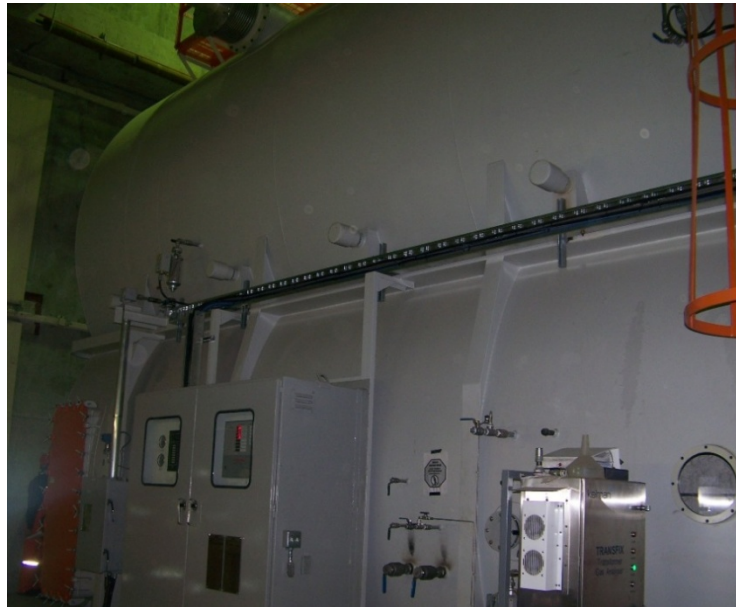
Photo 5 – Explosion-proof Enclosure for 230 kV/12 kV Transformer
