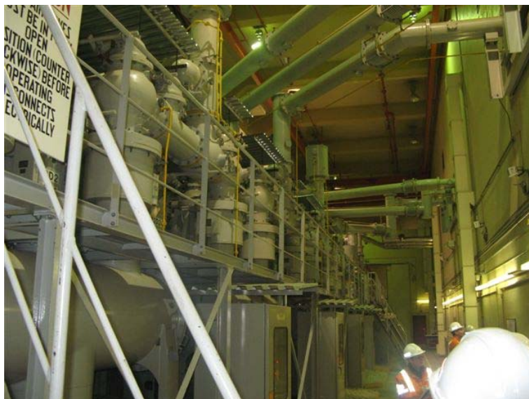
Photo 3 – Mitsubishi Lineup 230 kV GIS Switchgear
