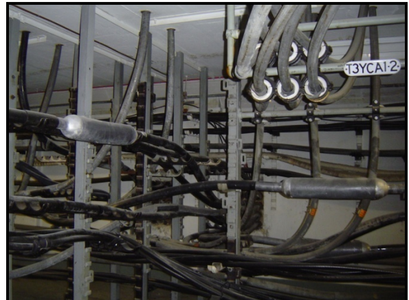
Figure 3: Windsor Station Cable Congestion
