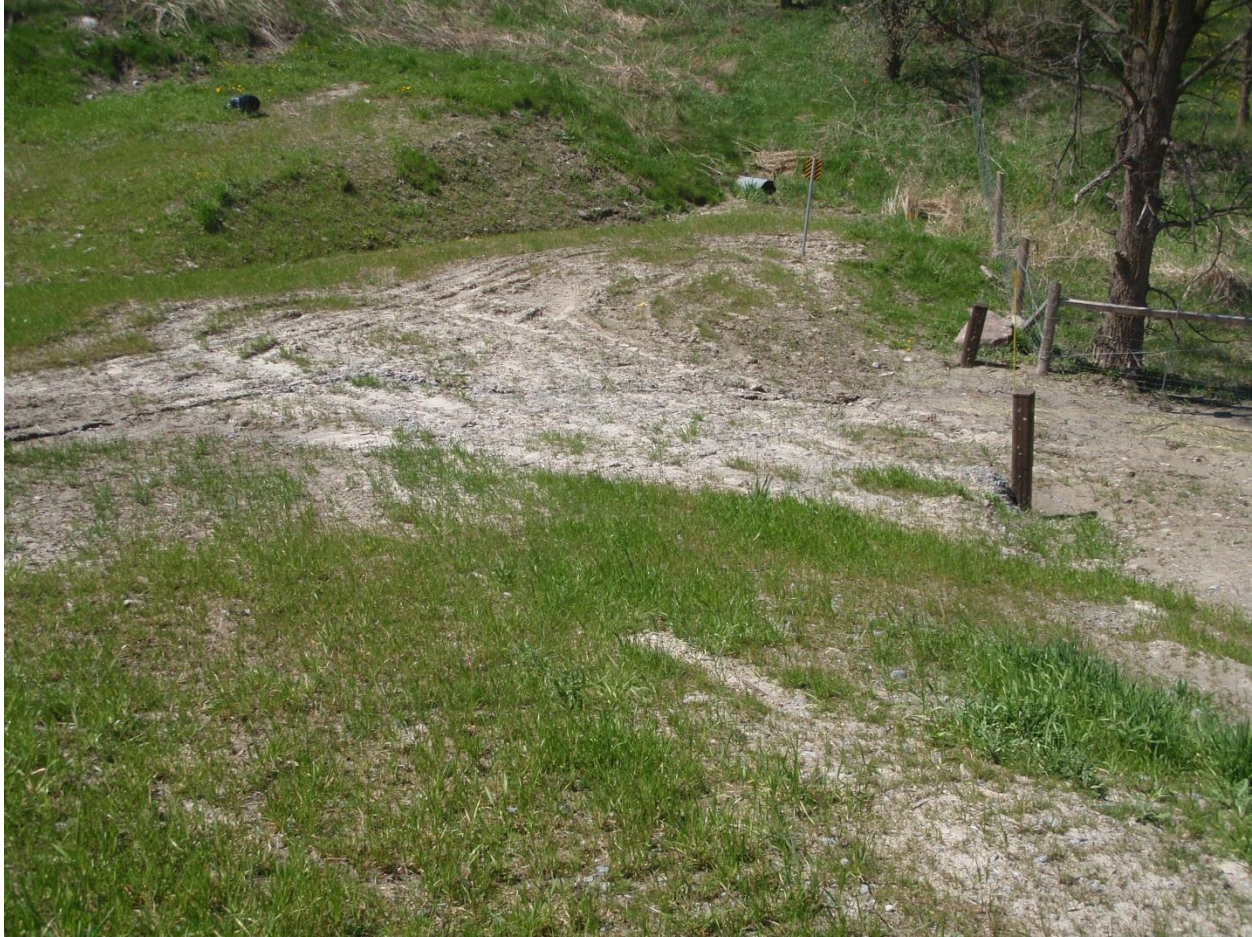
Photo 12 Poor vegetation establishment on a steep embankment on the the northwest intersection of the Davis Drive and Dufferin Street intersection (May 5, 2012)
