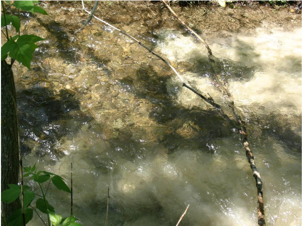
Photo 3 Close-up of drilling fluid release within the channel bed at WC5 (June 7, 2011)
