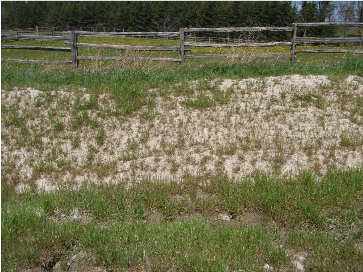
Photo 13 Poor vegetation establishment on the north backslope of Davis Drive, east of Dufferin Street (May 5, 2012)
