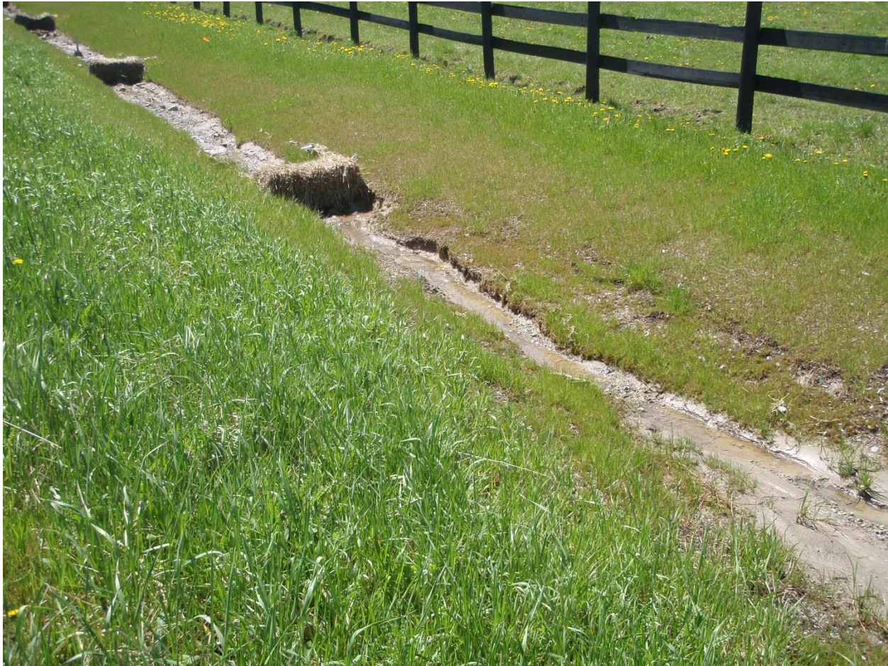
Photo 16 Erosion and sediment deposits southeast corner of the Jane Street and Davis Drive intersection (May 5, 2012)
