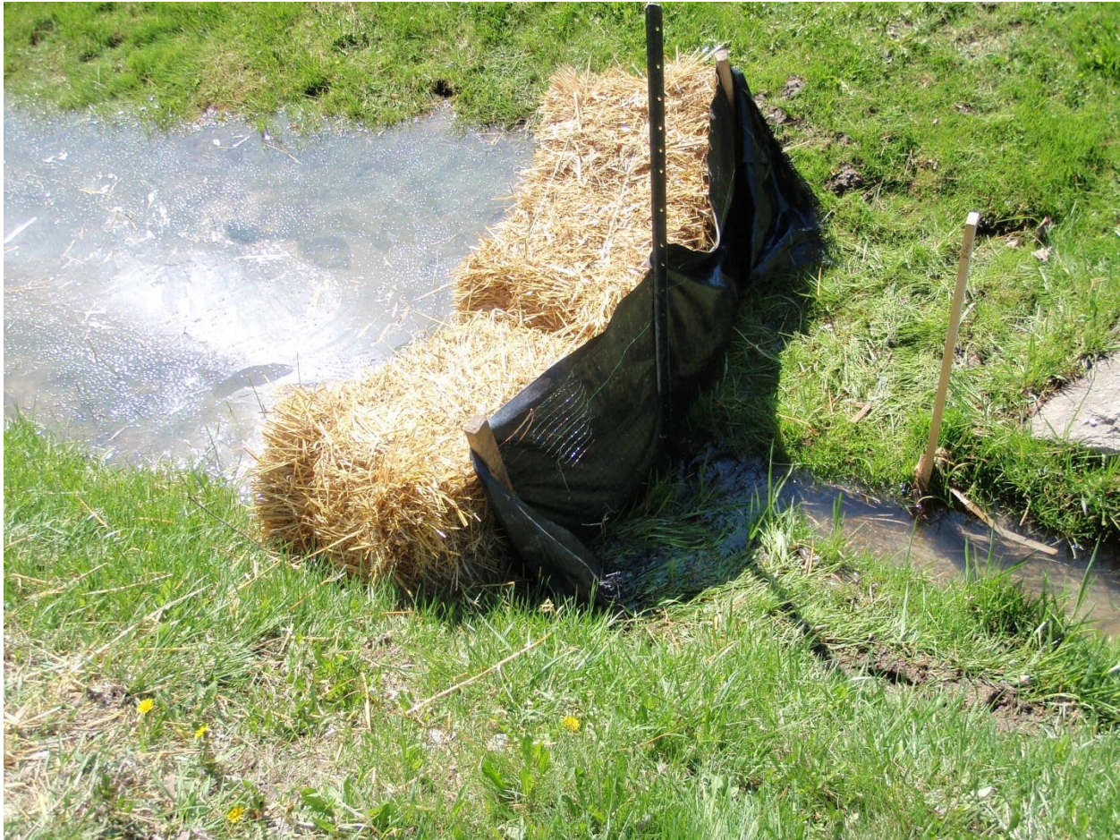
Photo 7 Check-dam installed in non-fisheries watercourse prior to drilling (drainage ditch) (May 7, 2011)
