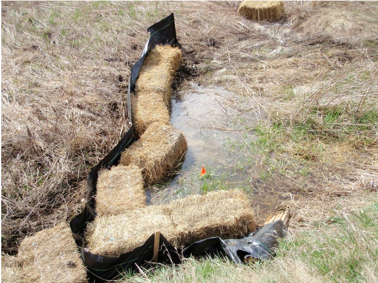
Photo 6 Sediment barrier adjacent watercourse installed prior to drilling (May 5, 2011)
