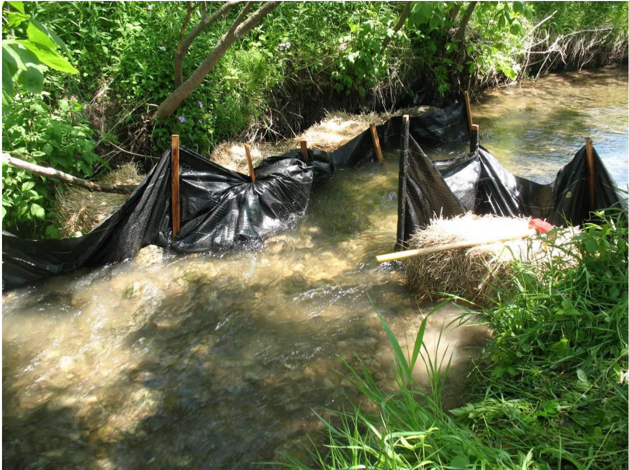
Photo 5 In-stream protection measures installed immediately after release to limit exposure of watercourse to drilling mud (June 7, 2011)
