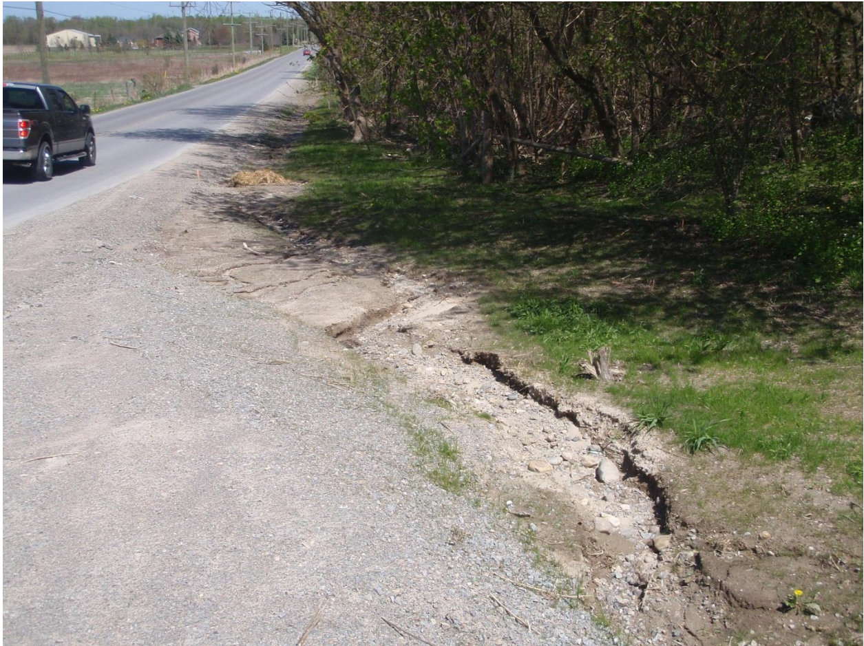
Photo 8 Surface erosion (gully) on ditch line on slope located on the east side of Dufferin Street, directly north of Miller's Side Road (May 5, 2012)
