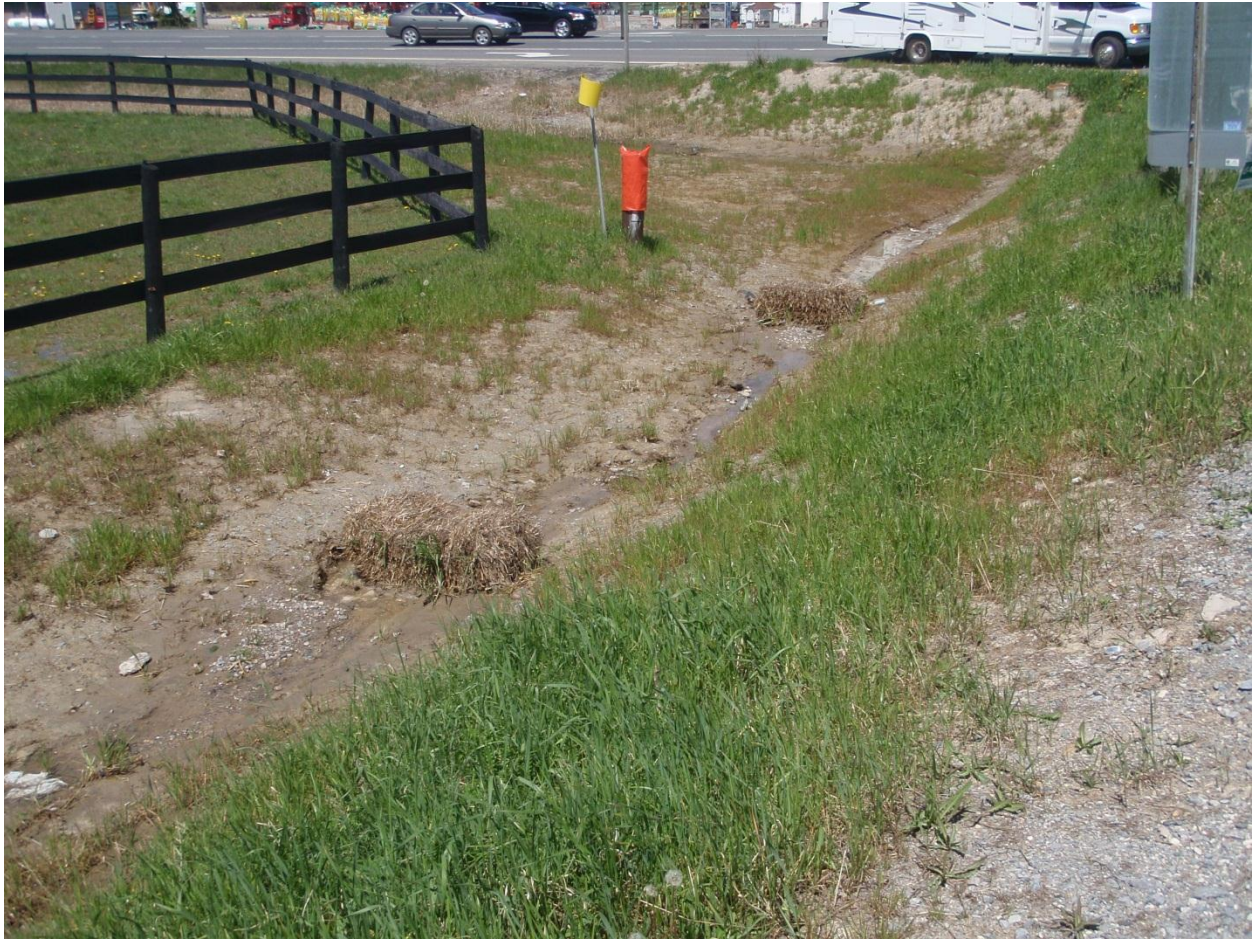
Photo 15 Erosion and sediment deposits southwest corner of the Jane Street and Davis Drive intersection (May 5, 2012)
