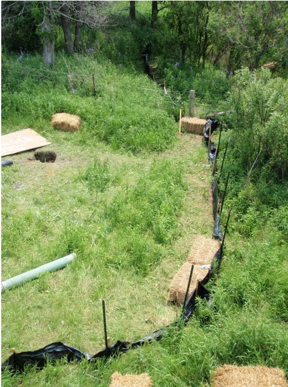
Photo 1 Erosion protection measures (silt fence and relief pit) setup up parallel to watercourse prior to drilling (June 7, 2011)
