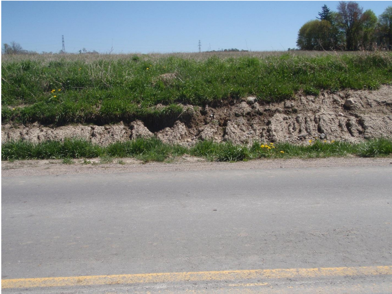
Photo 11 Slumping of road backslope on the east side of Dufferin Street, directly south of Miller's Side Road (May 5, 2012)
