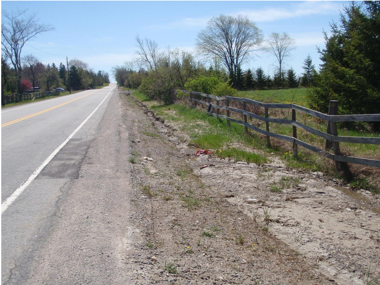
Photo 17 Erosion and sediment deposits east side of Jane Street (May 5, 2012)
