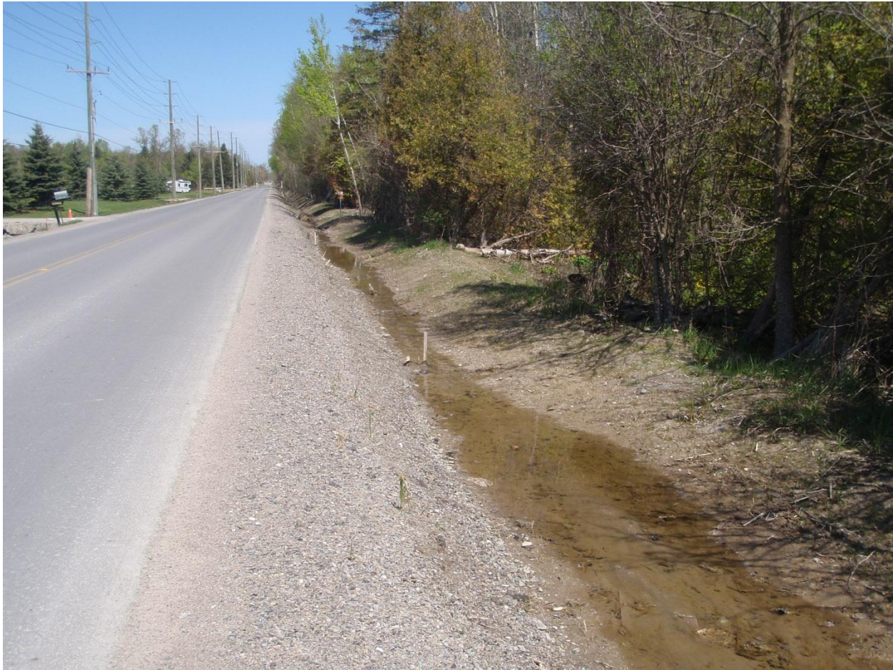
Photo 10 Poor vegetation establishment over excavated ditchline on the east side of Dufferin Street, South of the YEC (May 5, 2012)
