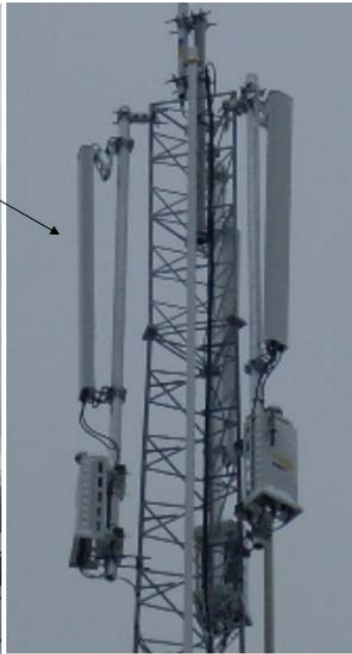
3-Sector WiMax Base Station (Base Station + Antenna's)
