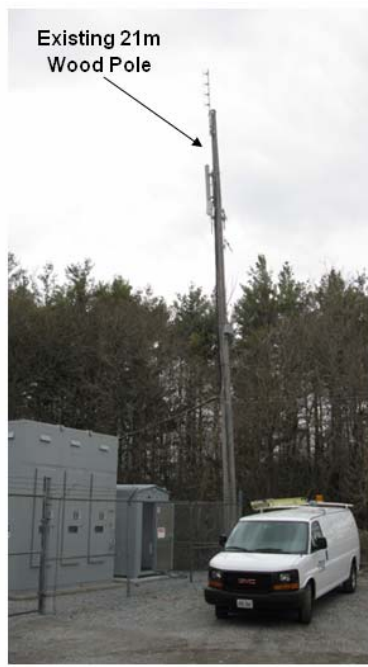
AMS4 - Aurora (Replace existing 21m Pole with 29.26m WiMax Tower)
