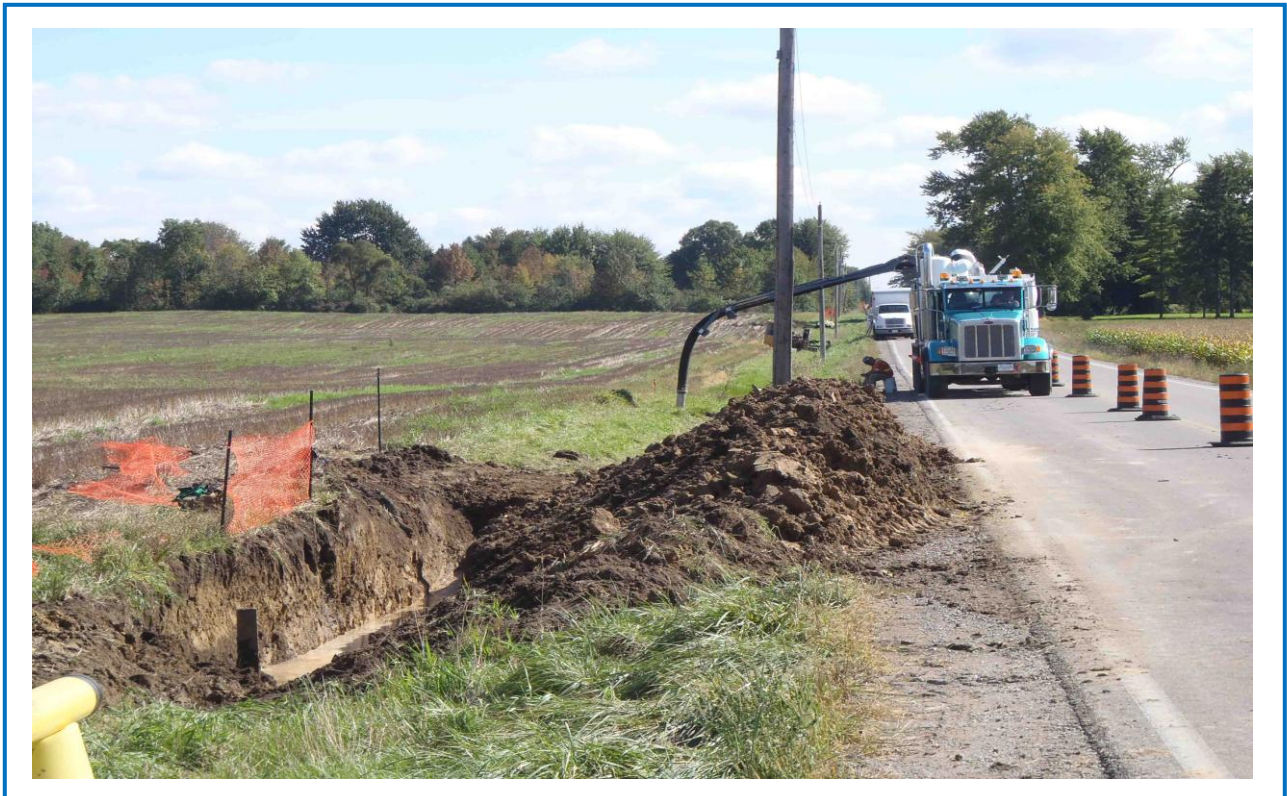
Along the pipeline right-of-way a vacuum truck was used to located other utilities prior to trenching or directional drilling.
