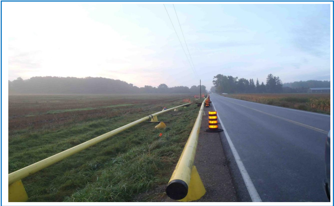
Prior to trenching operations the pipe was placed as far off the travelled portion of the road as possible and welded together.
