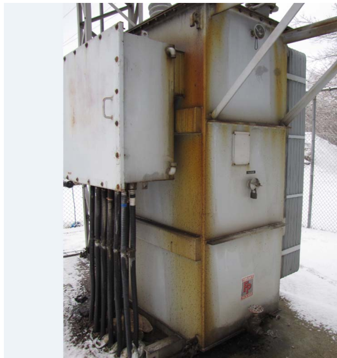
Figure 14: Oil leakage on a Distribution Transformer
