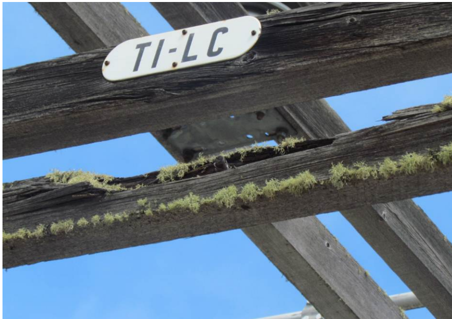
Figure 7 – Rotten Wooden Cross arm supporting live overhead equipment
