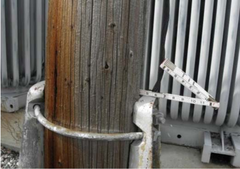
Figure 8 – 4” Deep Crack in Wood Supporting Structure
