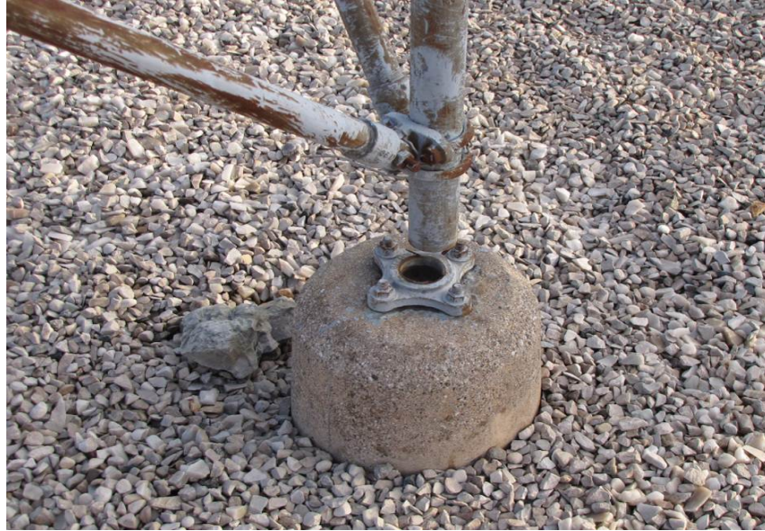
Figure 4 – Tube and Clamp Structure broken; supporting live overhead equipment
