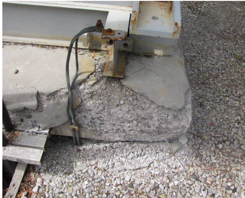
Figure 5 – Crumbling Concrete structure; supporting oil filled power transformer
