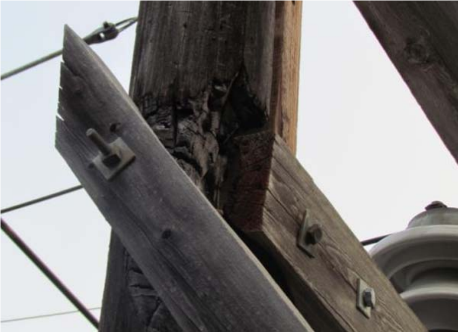
Figure 9 – Heavily Damaged Wood Supporting Structure
