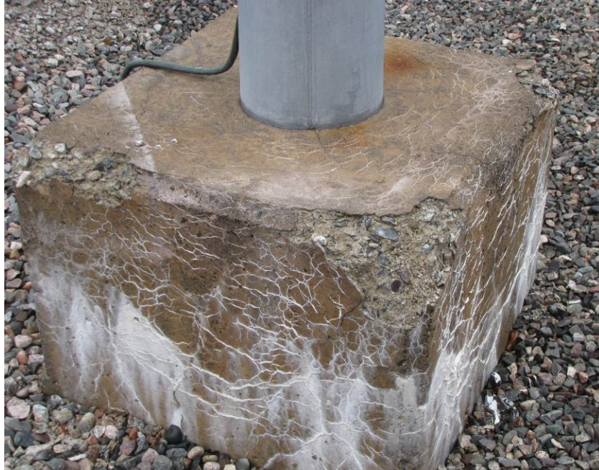
Figure 6 – Cracked Concrete foundation structure with live overhead equipment
