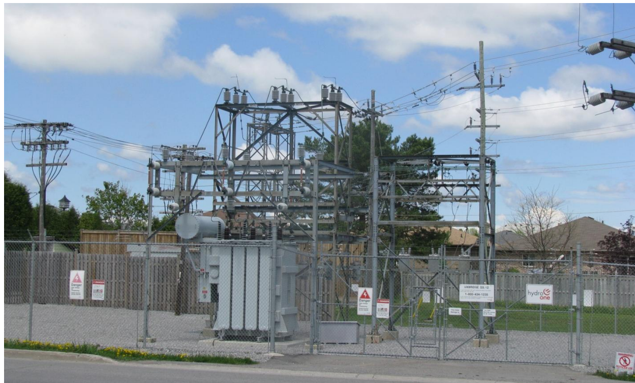
Figure 40: Typical Open Air Distribution Station
