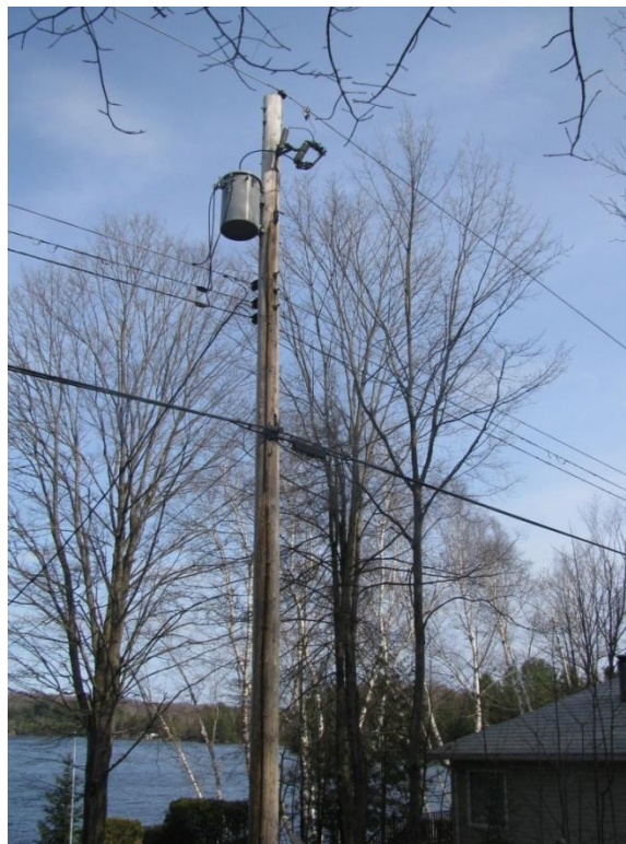
Figure 39: Typical Single Phase Pole-Top Transformer
