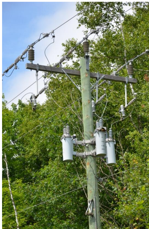
Figure 41: Single Phase Voltage Regulator (Left) and Three Phase Series Inductor (Right)
