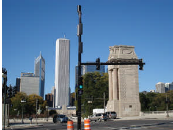
DAS equipment on traffic light pole near Grant Park
